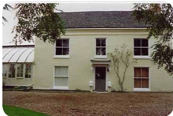
Rupert's Rest, Main Street, built about 1820, showing four-pane sash windows.
