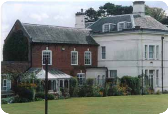
Glenn House, Church Road, showing the Georgian part of the house in orange/red brickwork and the later part of the building in off-white painted render.
