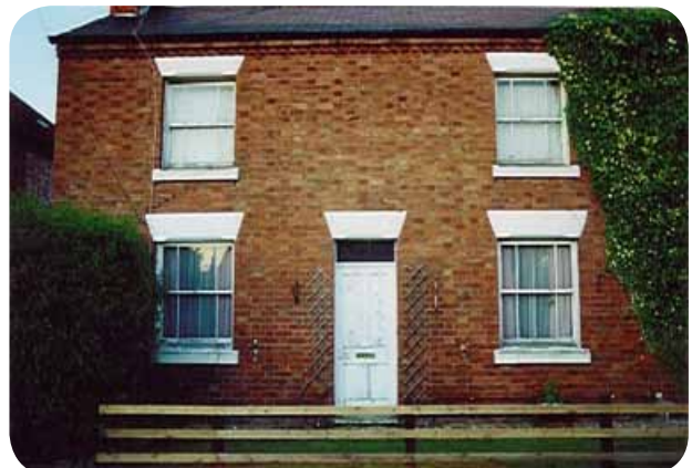
Double-fronted house, St. Thomas Road. Built about 1890, this house has stone lintels and windowsills, with brick detailing at the eaves.
