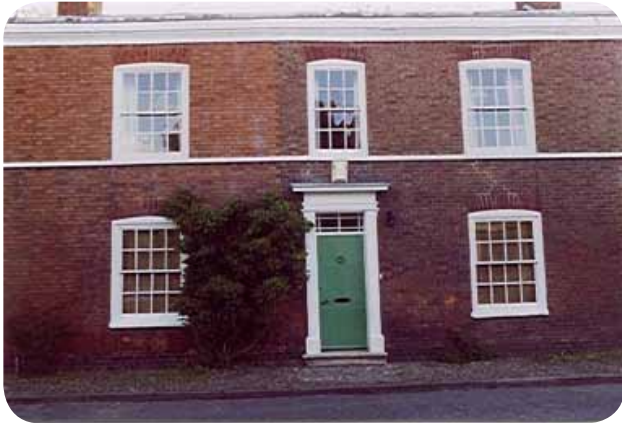
Bassets, No 3 The Nook. Built around 1800, extended about 1900.
