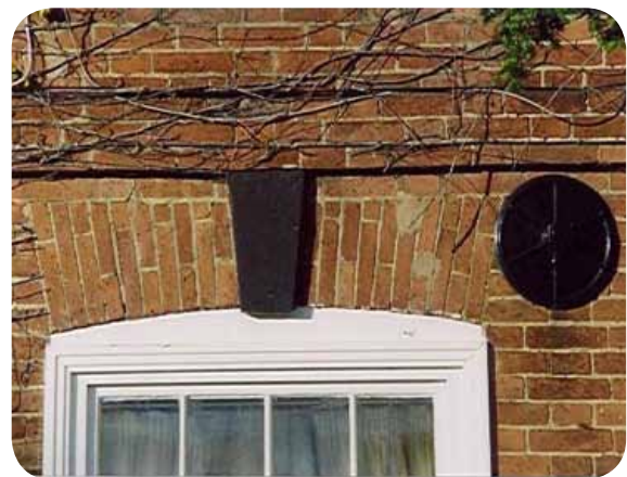
This detail from Trent House shows a cambered gauged brick lintel with painted keystones and a stringer of three courses of protruding brickwork above the window.
