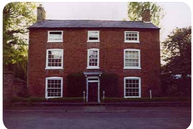
5 The Nook. Typical three-storey village house. Built around 1800
