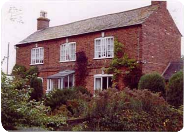
39 London Road, built around 1750. Casement windows have cambered lintels with keystones. Roofing is Swithland Slate.
