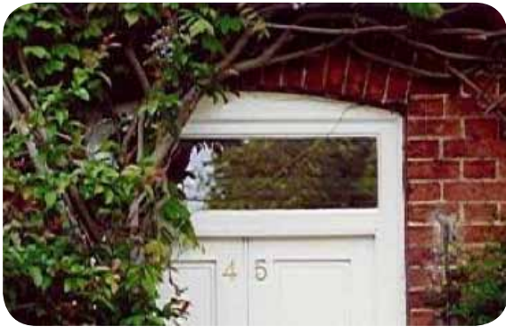
Chesterfield House, 45 Main Street, with cambered brick lintel above the main door.
