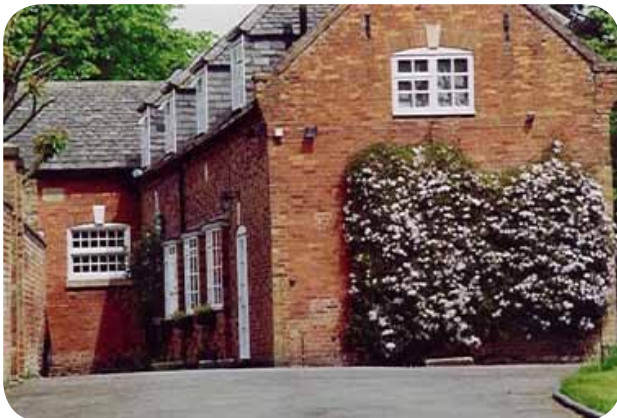
Tack House, Church Road. Conversion of former stabling built about 1800. Note cambered brick lintels with keystones.
