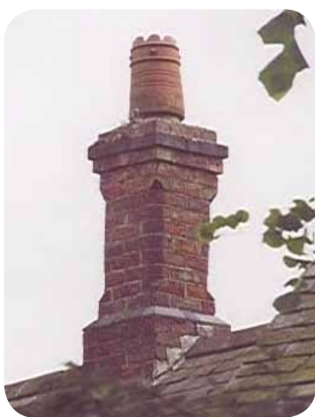
Small chimneystack at Wizards Haunt, 27 London Road
