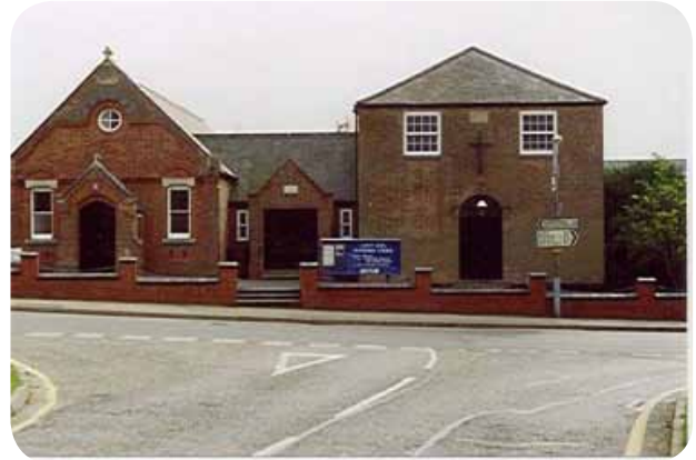
Great Glen Methodist Church. Built as a Wesleyan Chapel in 1827. Orange/red brickwork with Welsh Slate roof.
