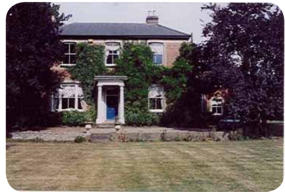
Mount Farm, London Road. Late Victorian double-fronted house showing Welsh Slate hipped roof.
