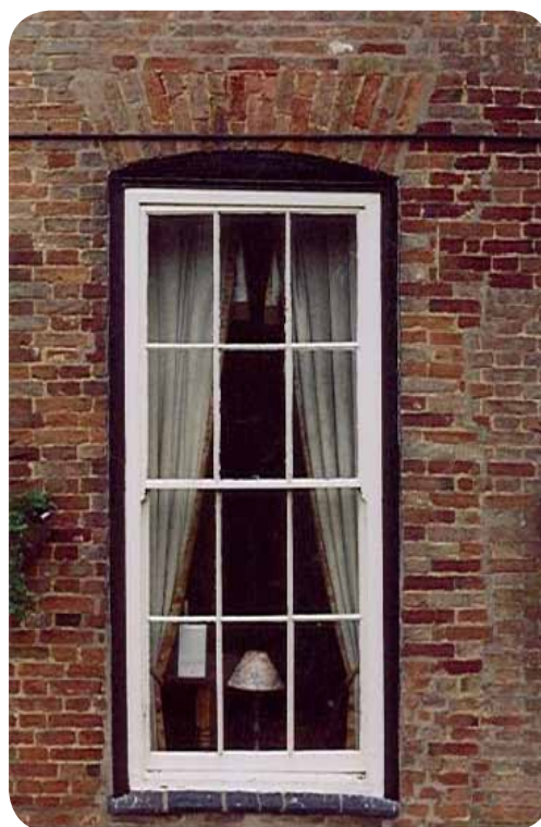
The Yews, London Road. Window detail showing twelve-pane sash window with gauged cambered brick lintel and windowsill made from "blue brick" tiles
