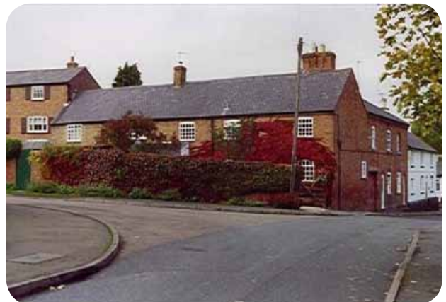
Cottages on High Street. Red brick with Welsh Slate roofs. Built around 1800
