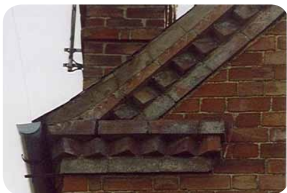
Victorian gable end detail, showing return feature in line with the eaves. The pattern continues along the front of the building below the gutter.
