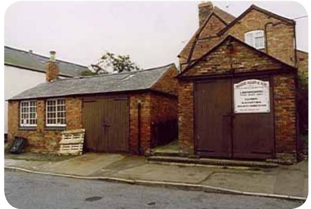
Old Forge, High Street. Cruck frame can be seen in the gable wall. Built around 1700 with many later additions.
