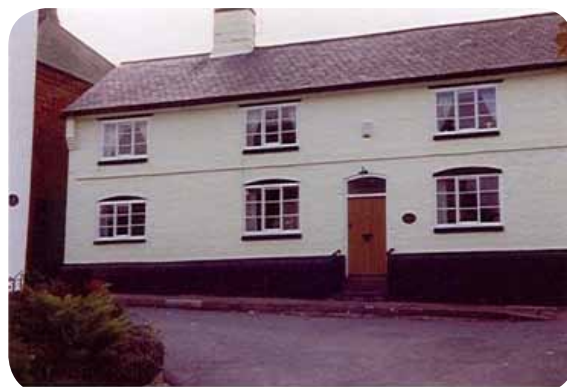
Glen Farmhouse, late 17th-century. Off-white paint hides the join in the brickwork where this house has been extended (left of the chimney). Note the three-course band of brickwork protruding above the first storey windows and the oak beams above the second storey windows.
