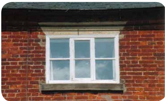
The Sycamores, 26 London Road. Attic window showing stone windowsill. Above the window the moulded brick cornice at the eaves is carried through the stone lintel.
