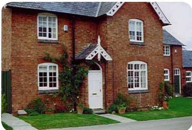
Cottage at Stretton Hall built around 1850. Note decorative fretwork fascia boards.
