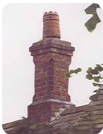
Small chimneystack at Wizards Haunt, 27 London Road
