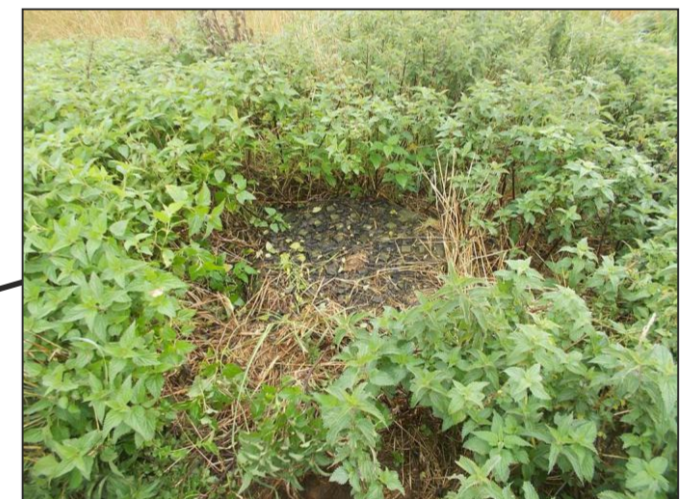
Inset 6 - Inspection manhole located along the decommissioned water collection infrastructure.
