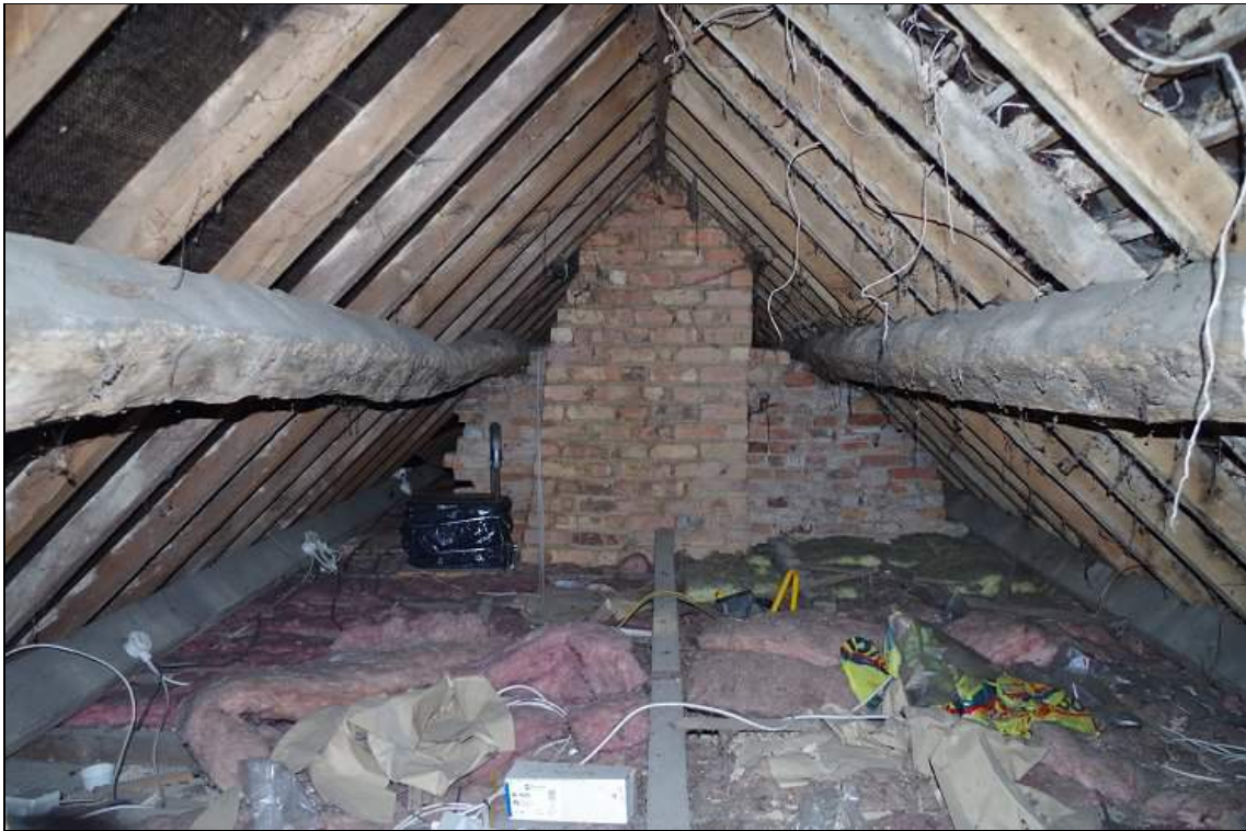
Photo 25. Roof structure over centre bay of East Range , empty mortices for wind braces are just visible in the upper face of the purlin on the left, towards either end, looking W.
