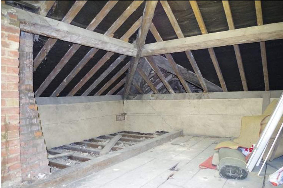
Photo 55. East attic room within Main Range , looking SE.
