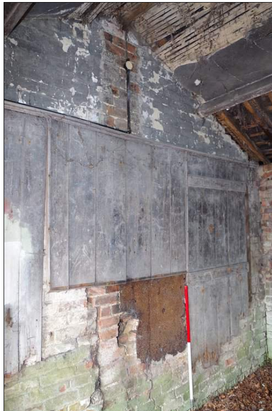
Photo 76. Matchboard on walls of Saddle Room and iron sheet behind stove, looking SW.
