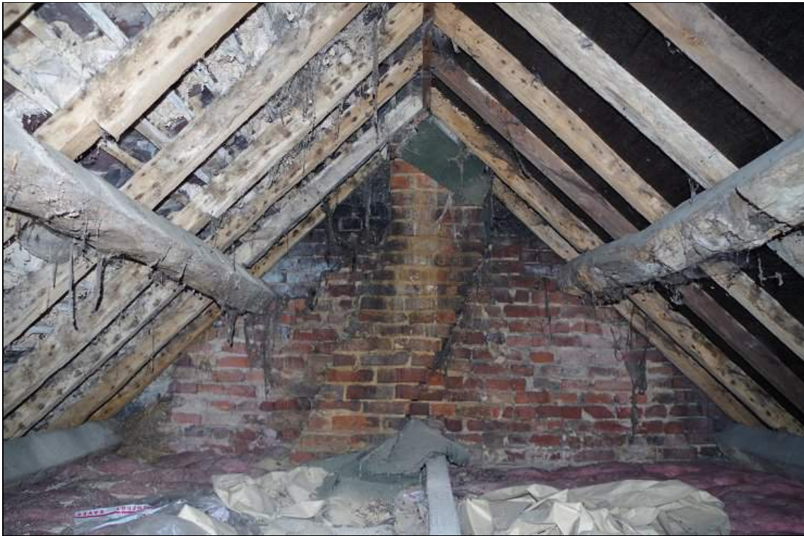
Photo 23. Roof space over E bay of East Range , note lap dovetail matrix in purlin on right.
