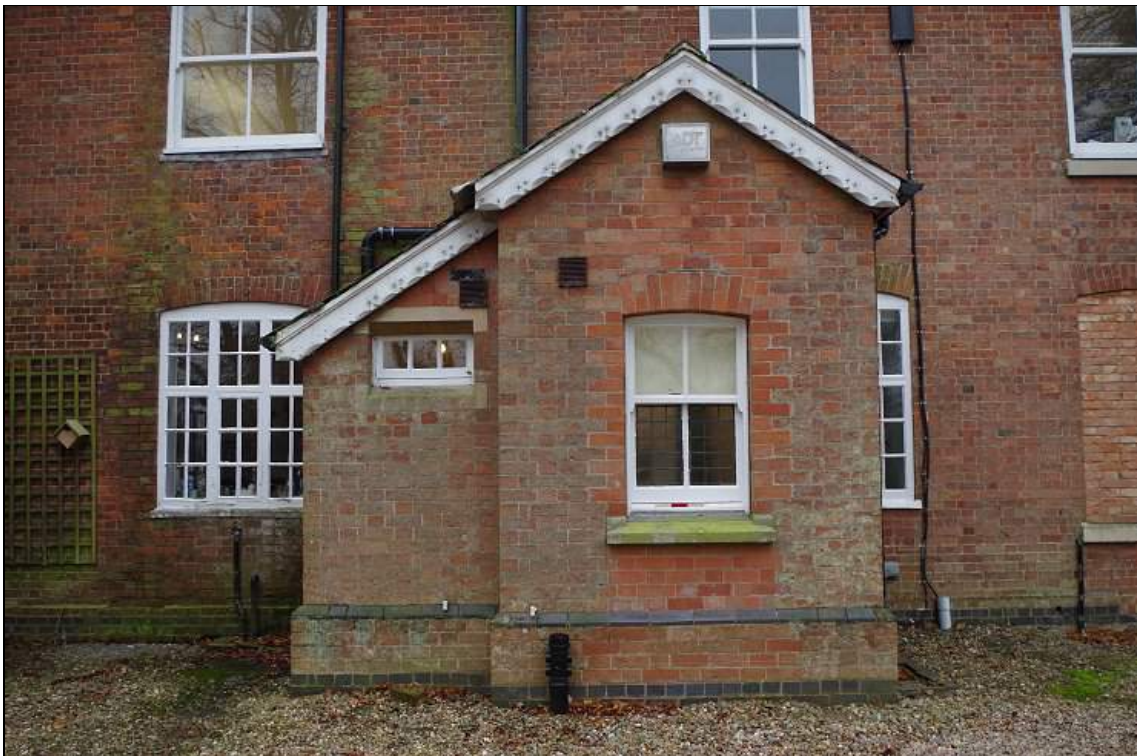
Photo 72. North Wing showing former doorway converted into window, looking S.
