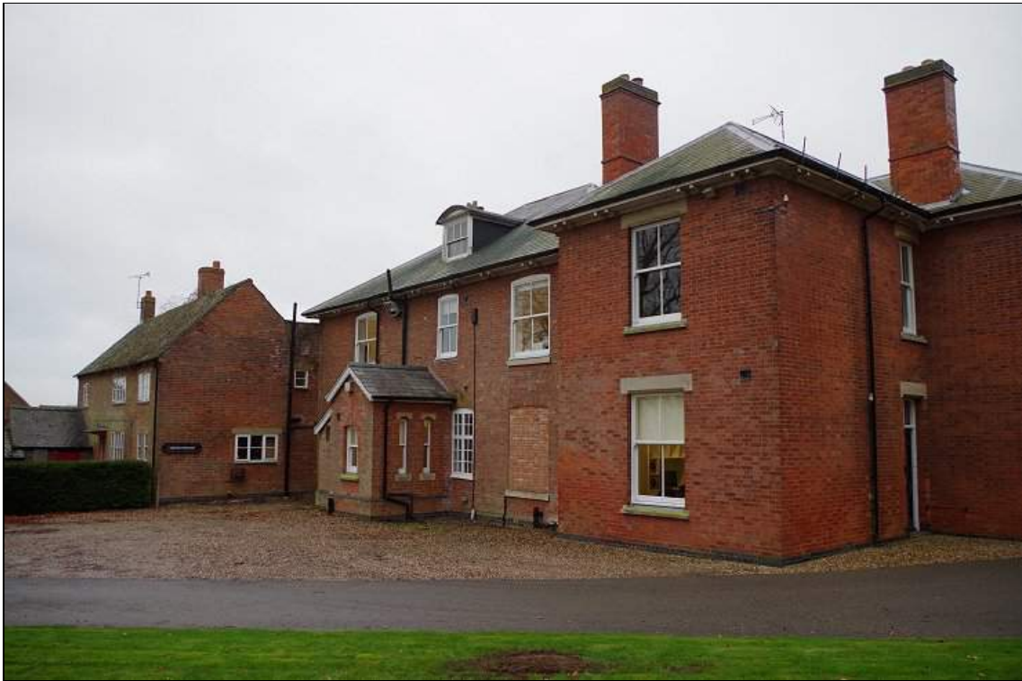
Photo 3. General view of Bittesby House from the NW.
