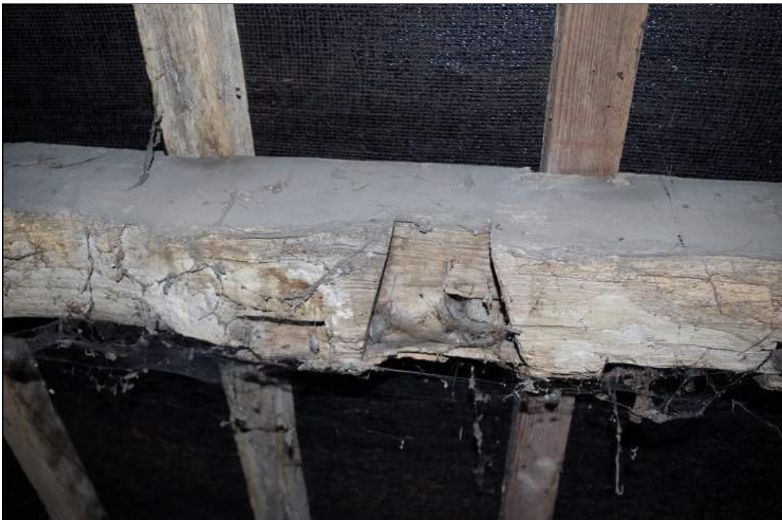
Photo 24. Wall plate re-used as purlin in roof of East Range , with empty lap dovetail matrix for tie-beam and birds-mouths for rafters.
