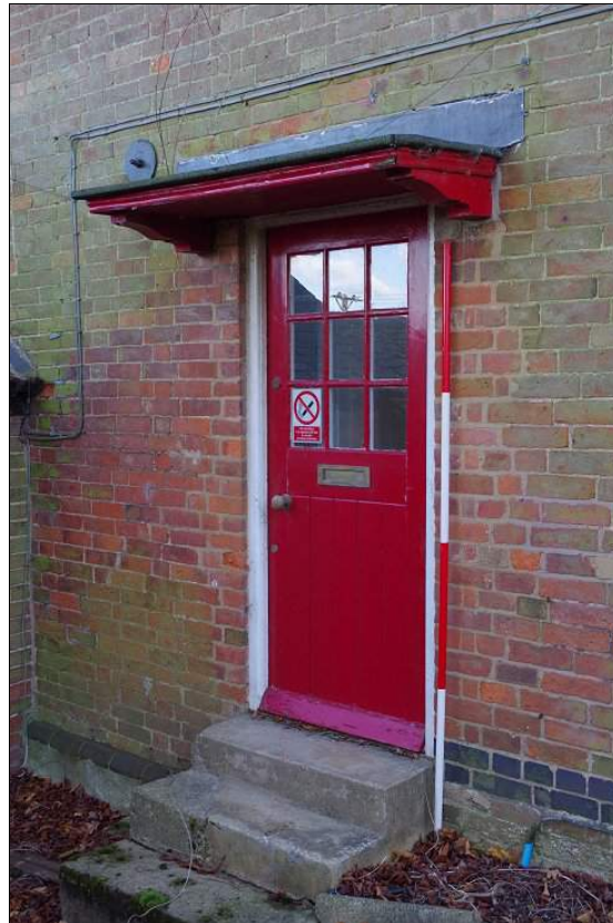
Photo 22. North front door and canopy of East Range , looking SE.
