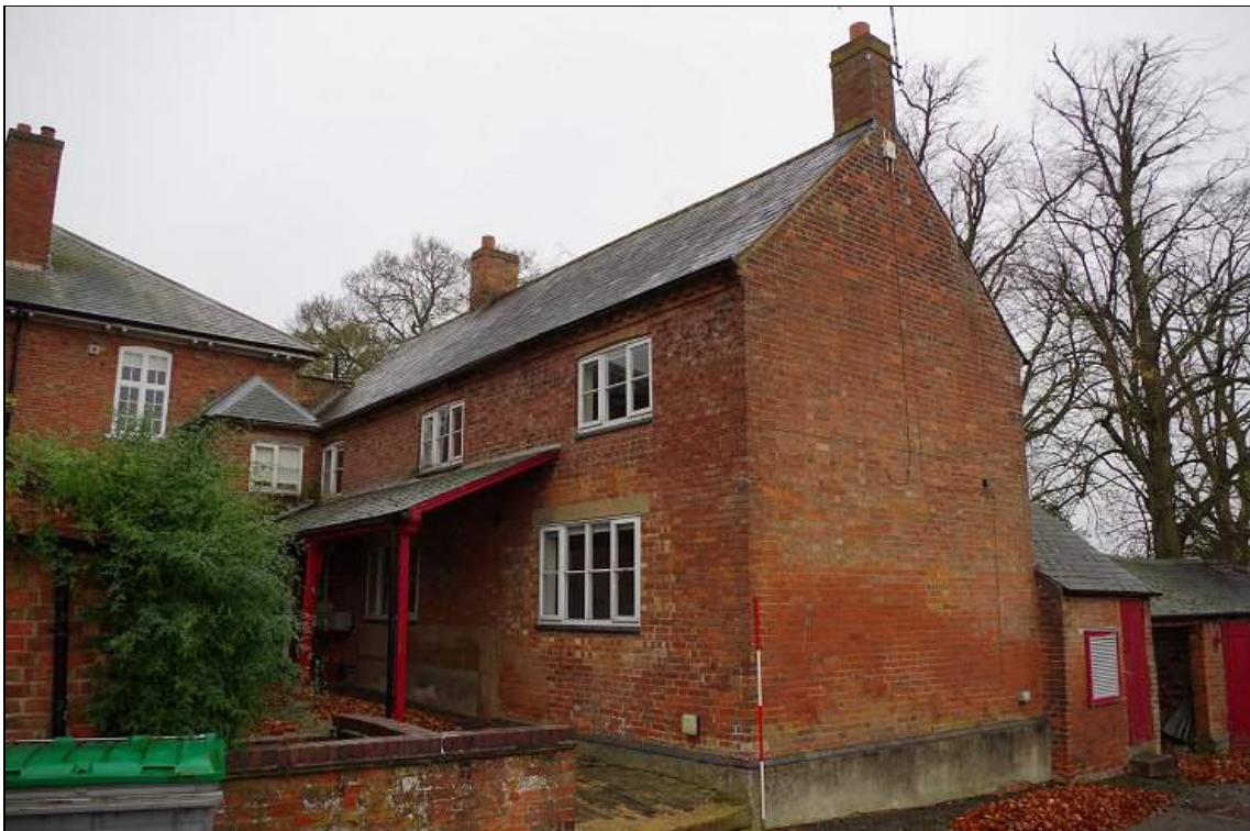
Photo 6. East Range of Bittesby House from the SE.
