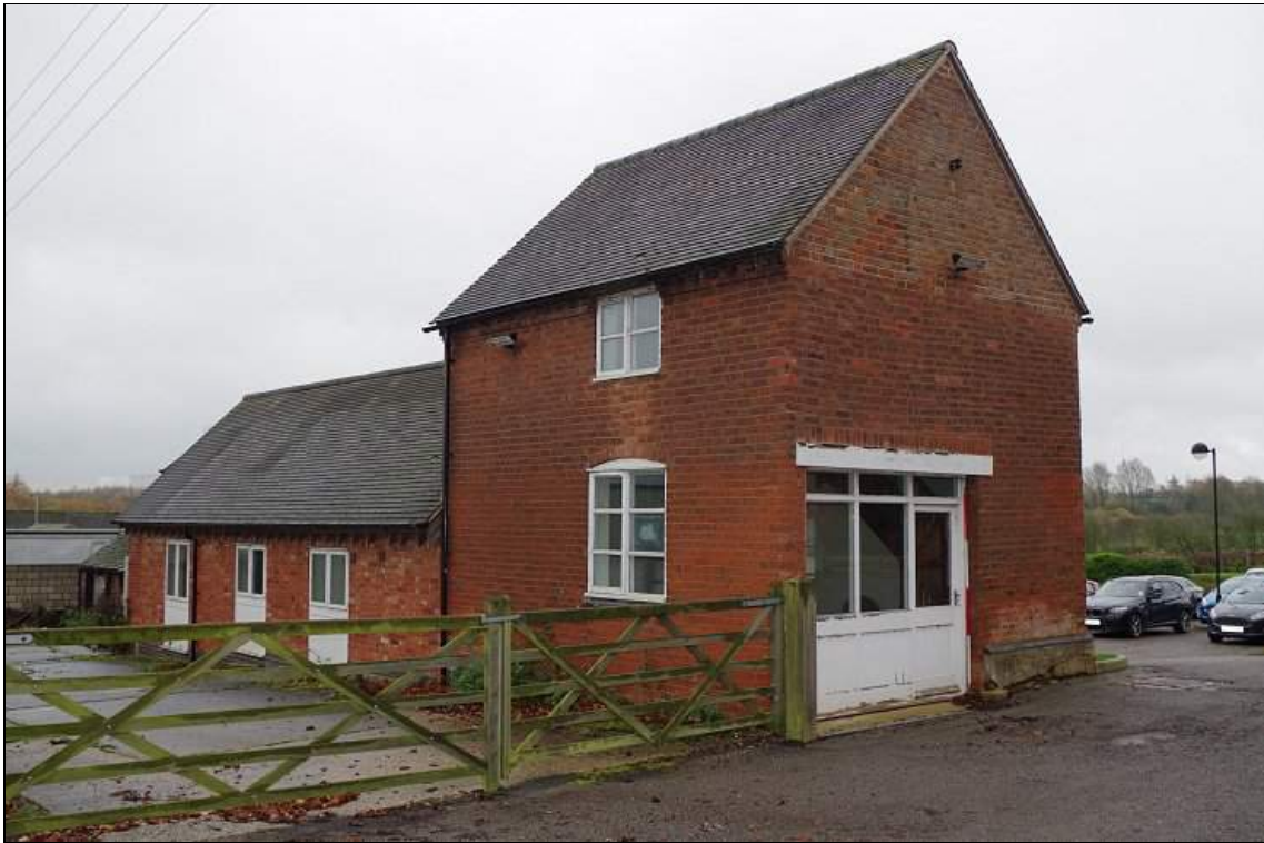
Photo 83. Barn with Granary Over & Cow House noted in 1944 Sale Particulars, looking SE.
