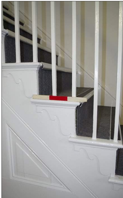
Photo 34. Detail of shaped tread ends to staircase within Main Range .
