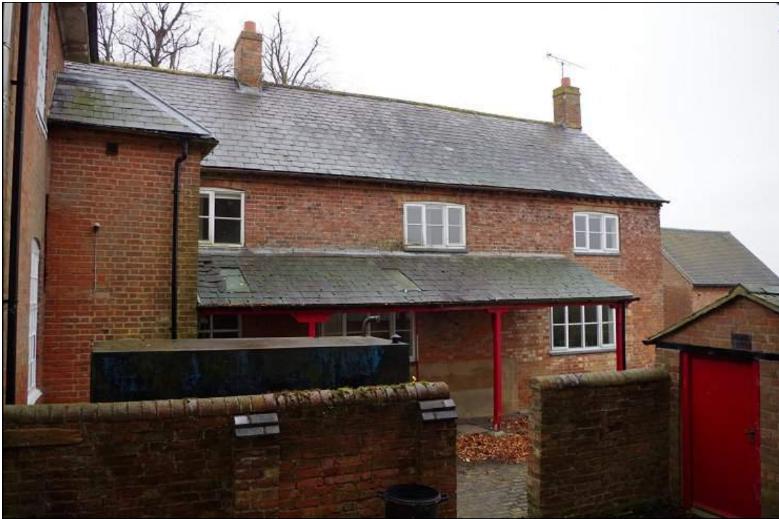
Photo 7. South elevation of the East Range , looking NNE.
