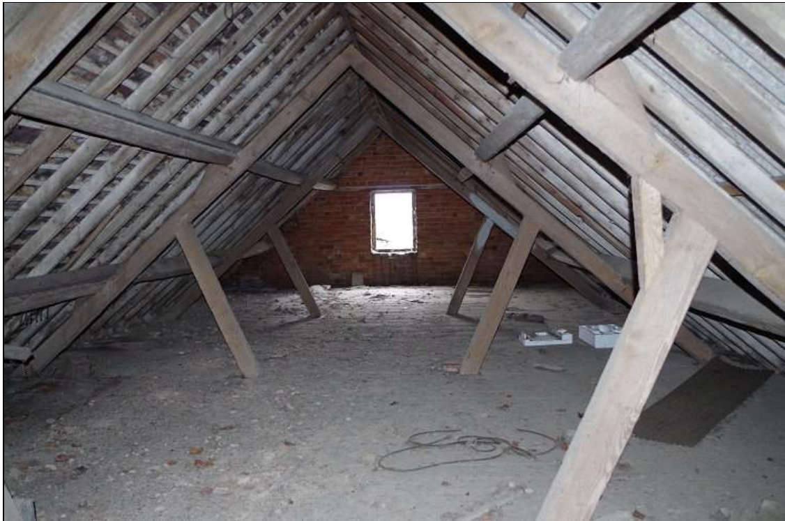
Photo 91, Granary over Workshop , looking E.
