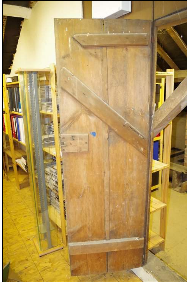
Photo 53. Door into west attic room within Main Range , looking SW.
