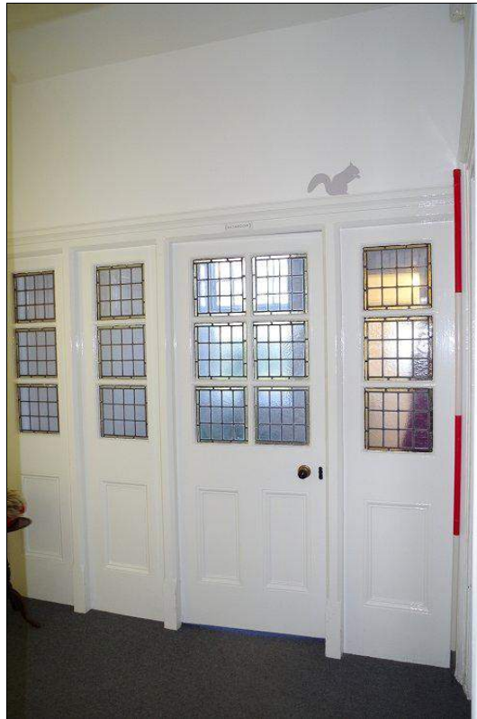
Photo 39. Glazed timber partition within back hall of Main Range , looking N.
