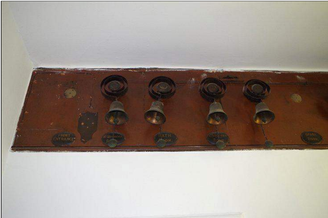
Photo 41. Detail of servant call bells in back hall of Main Range .
