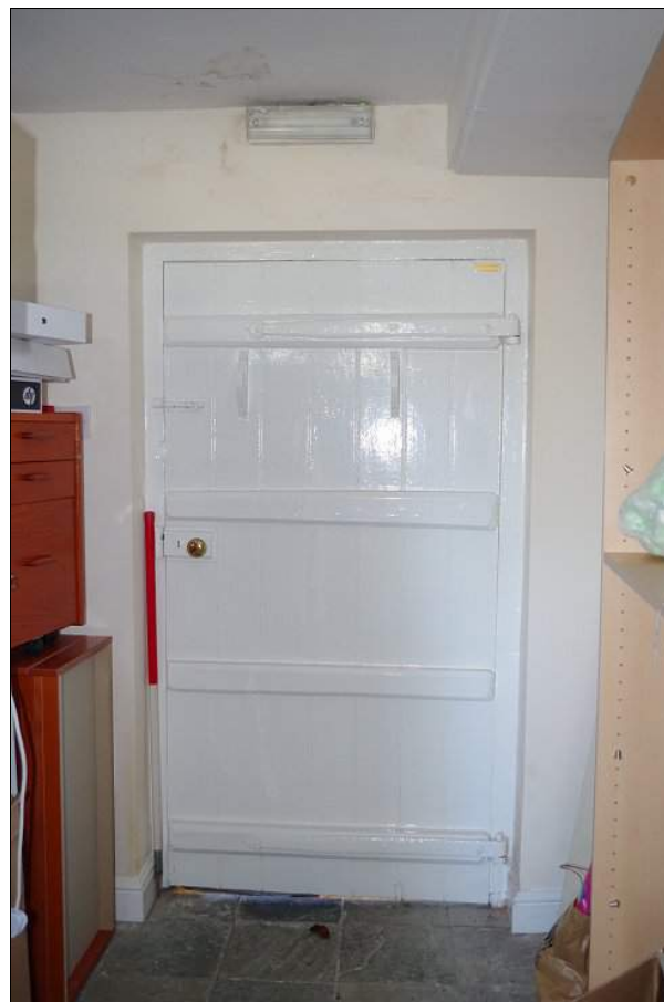
Photo 14. Door in S wall of W room of East Range opening into Rear Porch , looking N.
