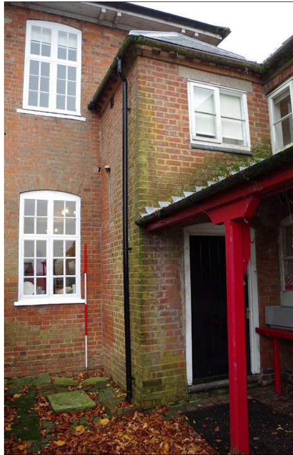
Photo 61. The Rear Porch linking Main Range (left) and East Wing (right), looking NW.
