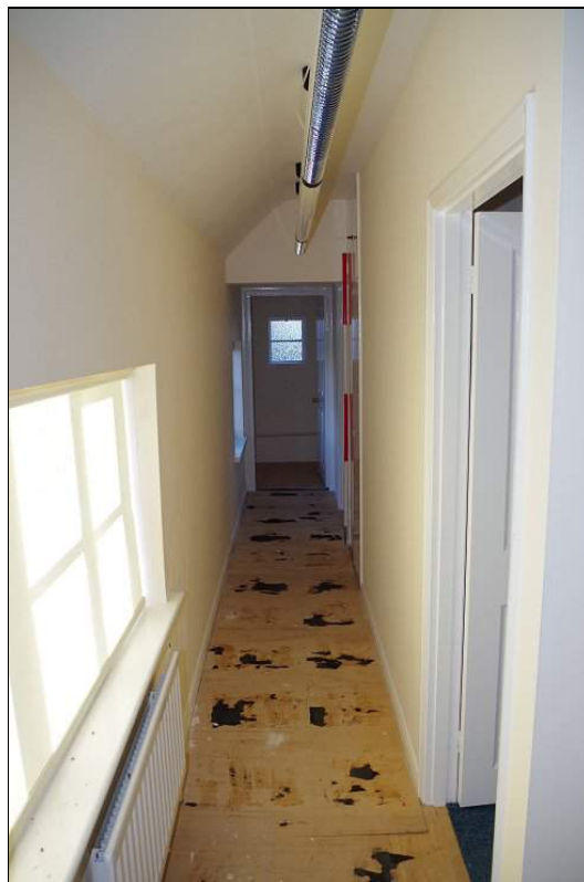
Photo 16. View W along first floor corridor on S side of East Range .
