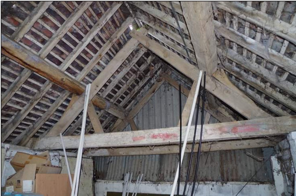
Photo 80. Roof structure of Three-stall Nag Stable range, looking NE.
