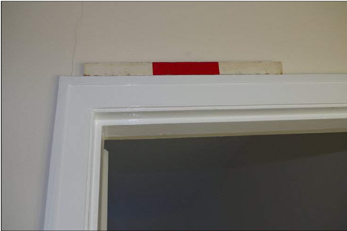
Photo 21. Detail of 1930s style doorframe within East Range .
