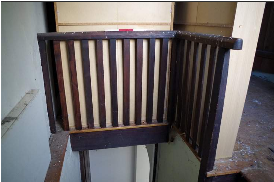
Photo 52. Balustrade around top of attic staircase within Main Range , looking S.
