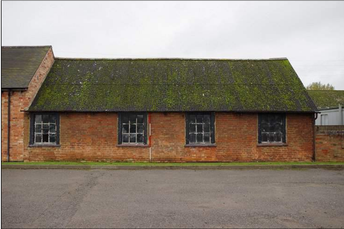
Photo 89. South elevation of Workshop noted in 1944 Sale Particulars, looking N.
