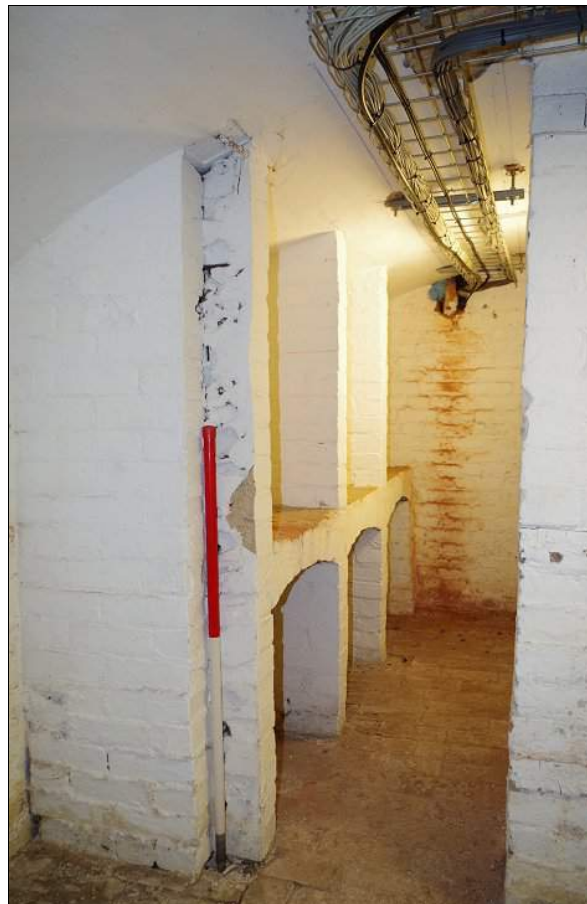
Photo 60. Smaller cellar room below Main Range with wine storage bins, looking N.
