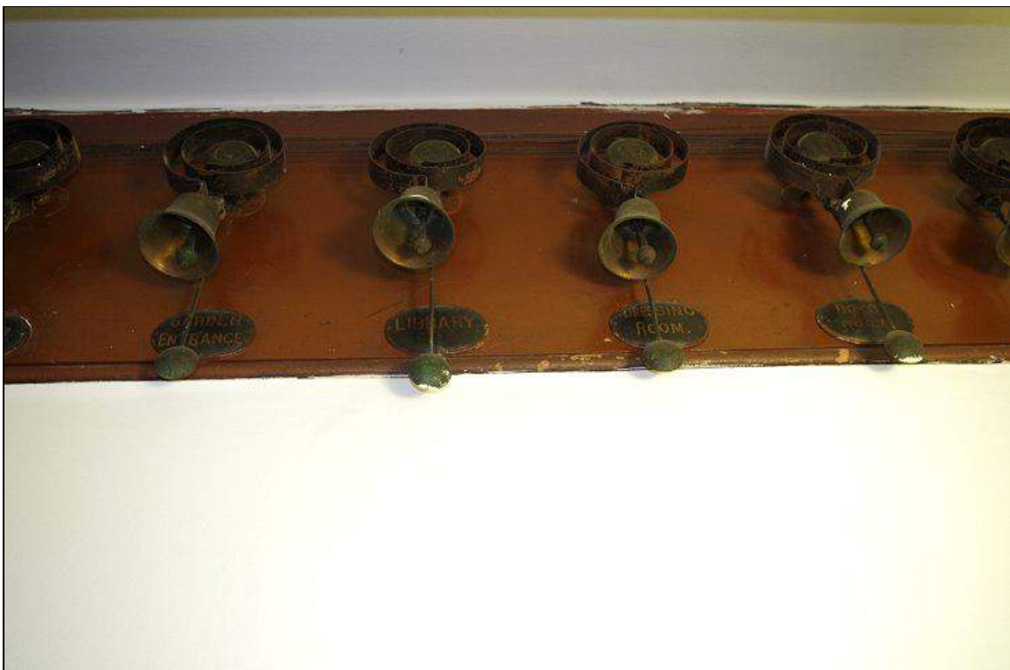
Photo 42. Detail of servant call bells in back hall of Main Range .
