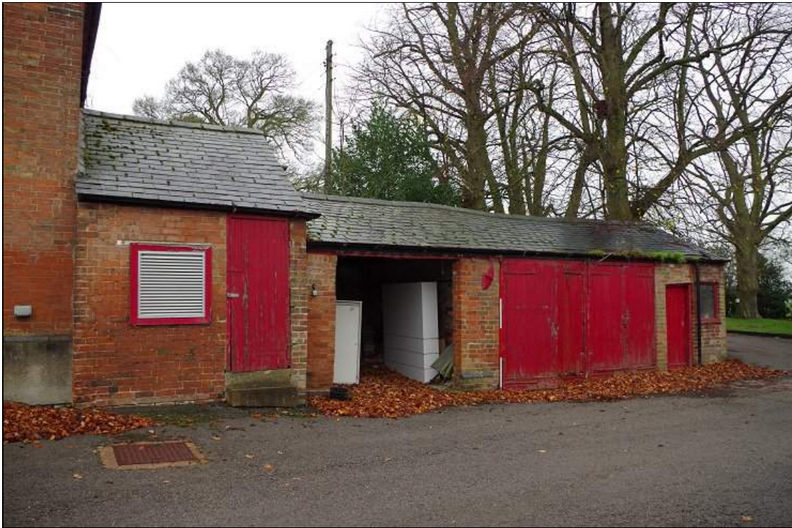
Photo 73. From left to right: Coal Place, Garage and Saddle Room noted in 1944 Sale Particulars, looking W.
