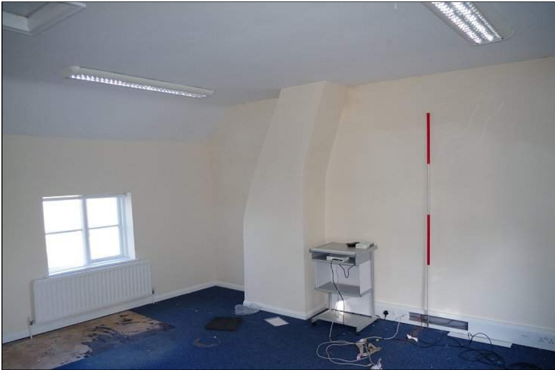
Photo 17. First floor E room within East Range , looking NE (note roof access hatch).
