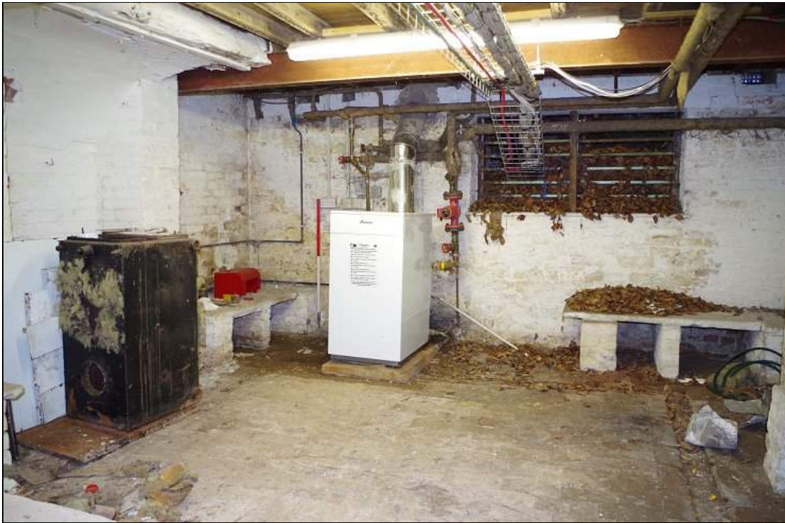
Photo 59. Larger cellar room at SE corner of Main Range , looking E.
