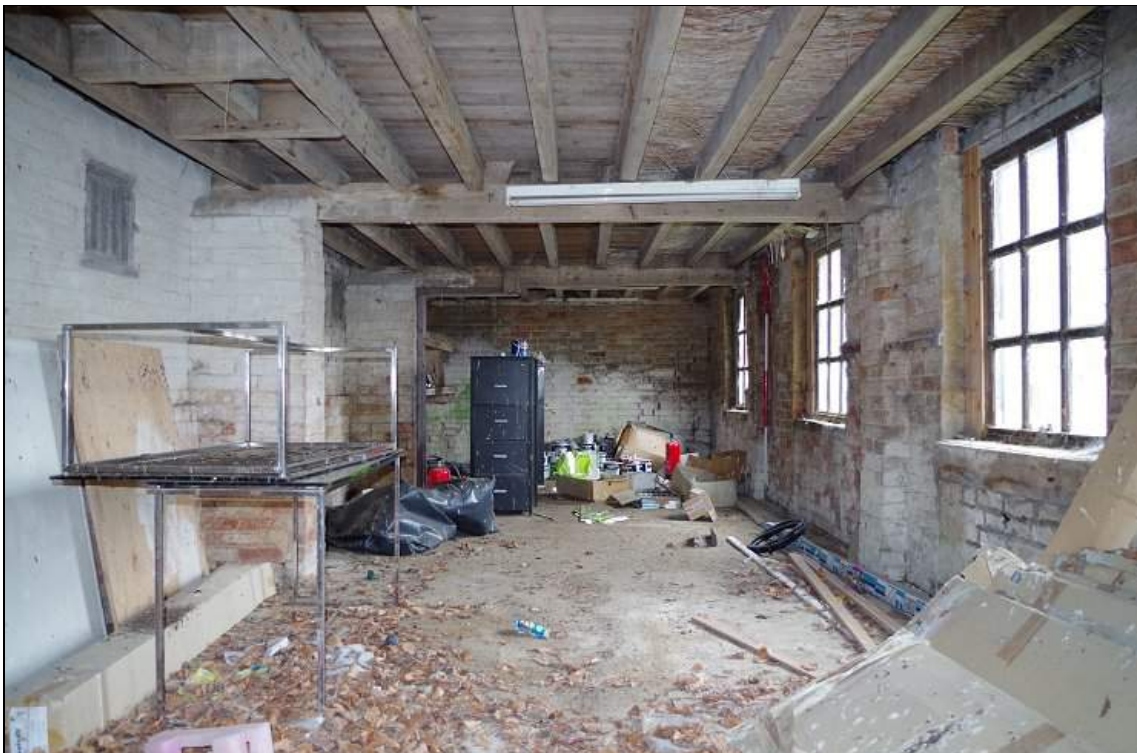
Photo 90. Interior of Workshop , looking E.
