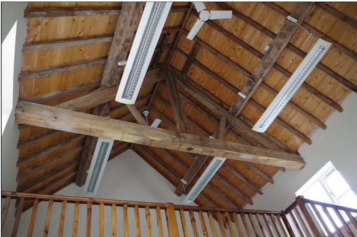
Photo 84. King-post truss supporting roof of Barn with Granary Over , looking E.
