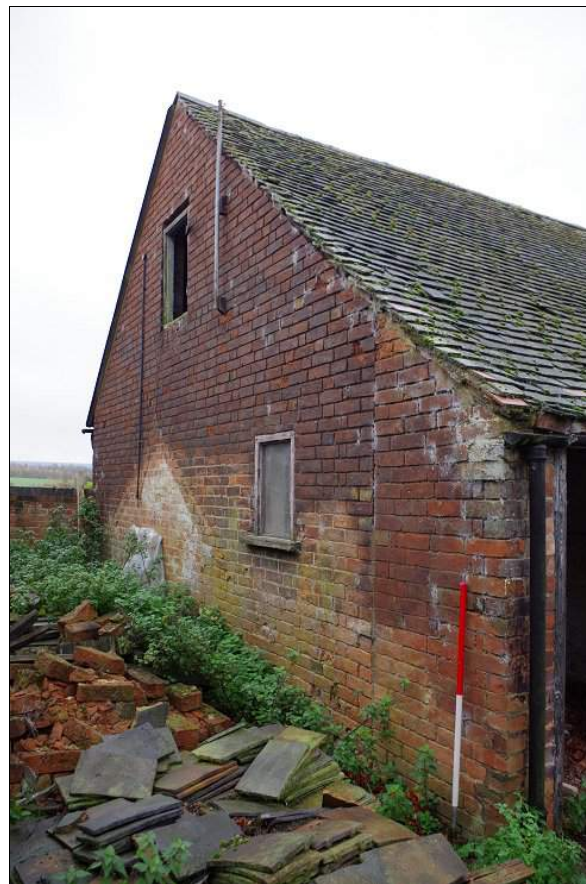
Photo 92. Constructional break between Workshop and later Pig Sties or Calf Places plus outline of former Pig Sties adjoining E end of Workshop , looking SSW.
