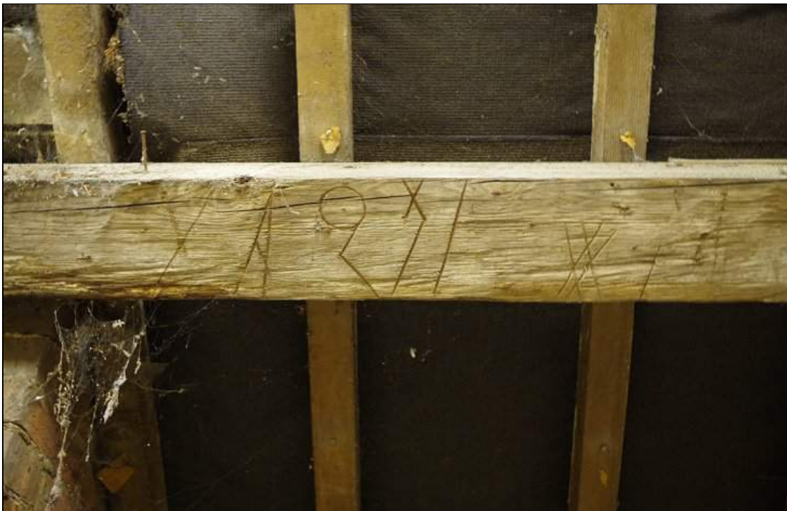
Photo 58. Shipping marks on roof purlin within Main Range .
