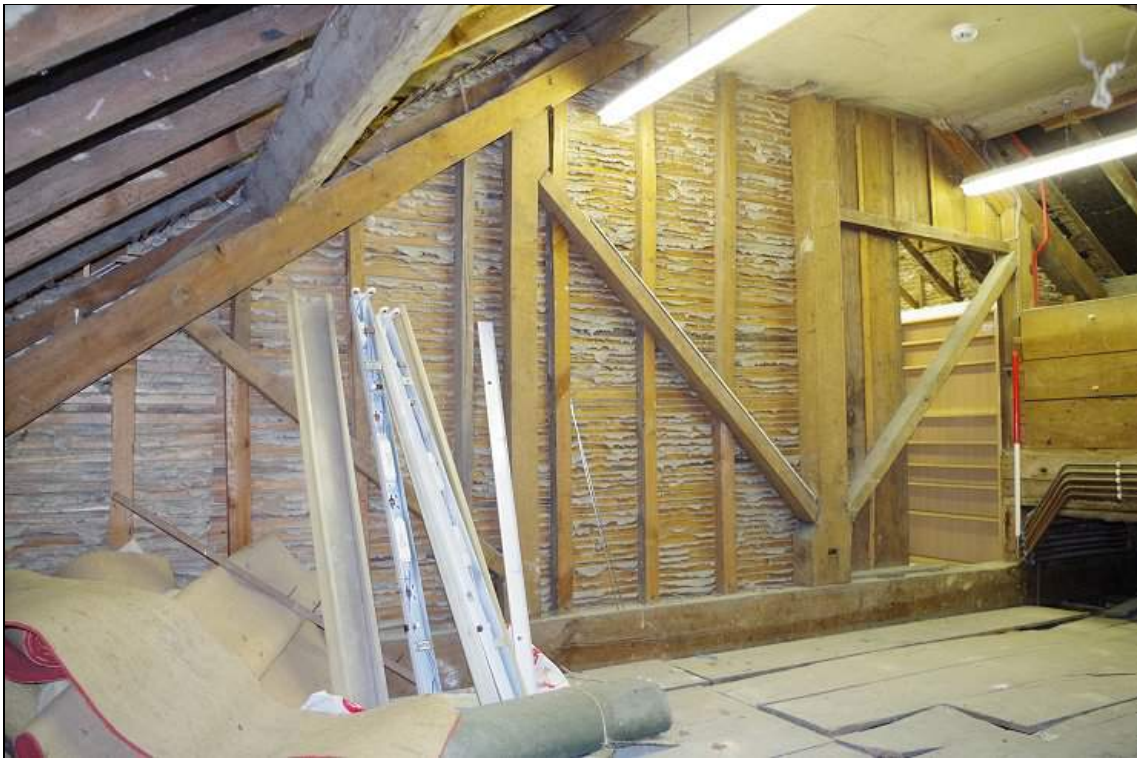
Photo 54. East attic room within Main Range , showing king-post roof truss, looking NW.
