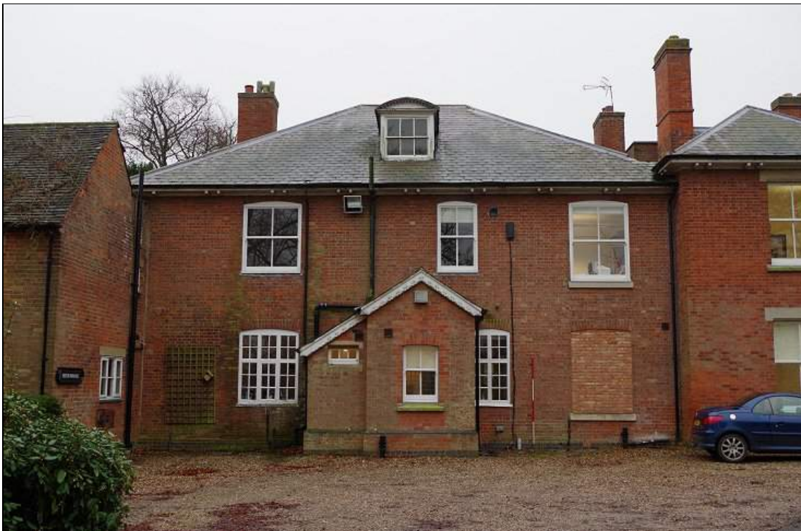
Photo 28. North elevation of Main Range , looking S.
