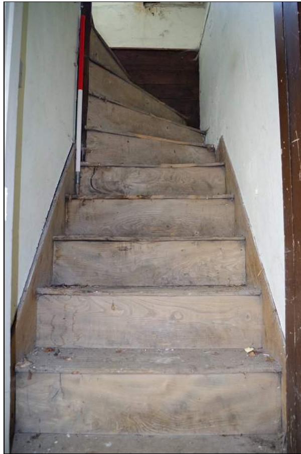
Photo 51. Attic staircase within Main Range , constructed from elm, looking N.
