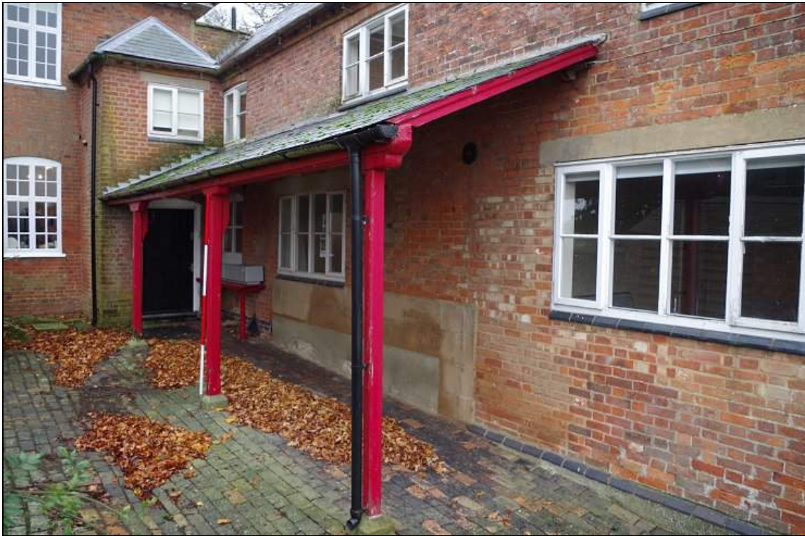
Photo 9. S elevation of East Wing (right), covered Lean-to and Rear Porch , looking NW.
