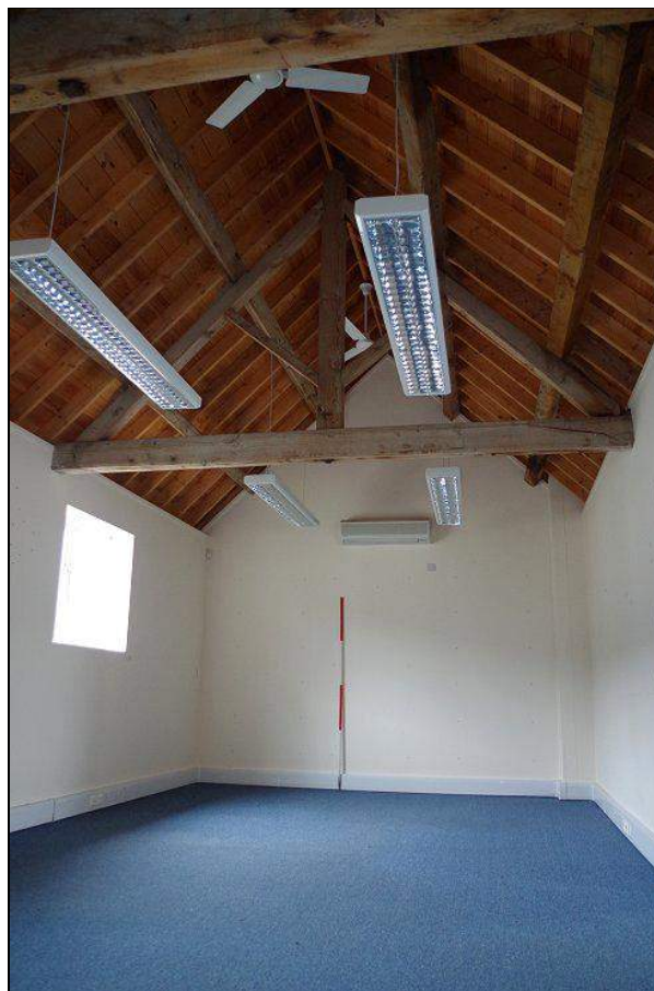
Photo 86. Interior of former Cow House showing king-post roof trusses, looking E.
