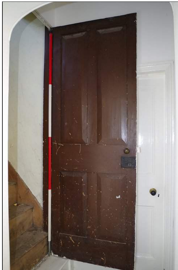
Photo 50. Doorway in rear corridor of Main Range leading to attic staircase, looking E.
