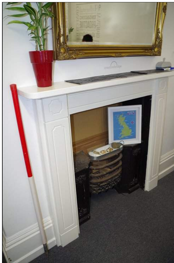
Photo 46. Fireplace in SE bedroom with stone/slate surround and hob grate, looking NE.
