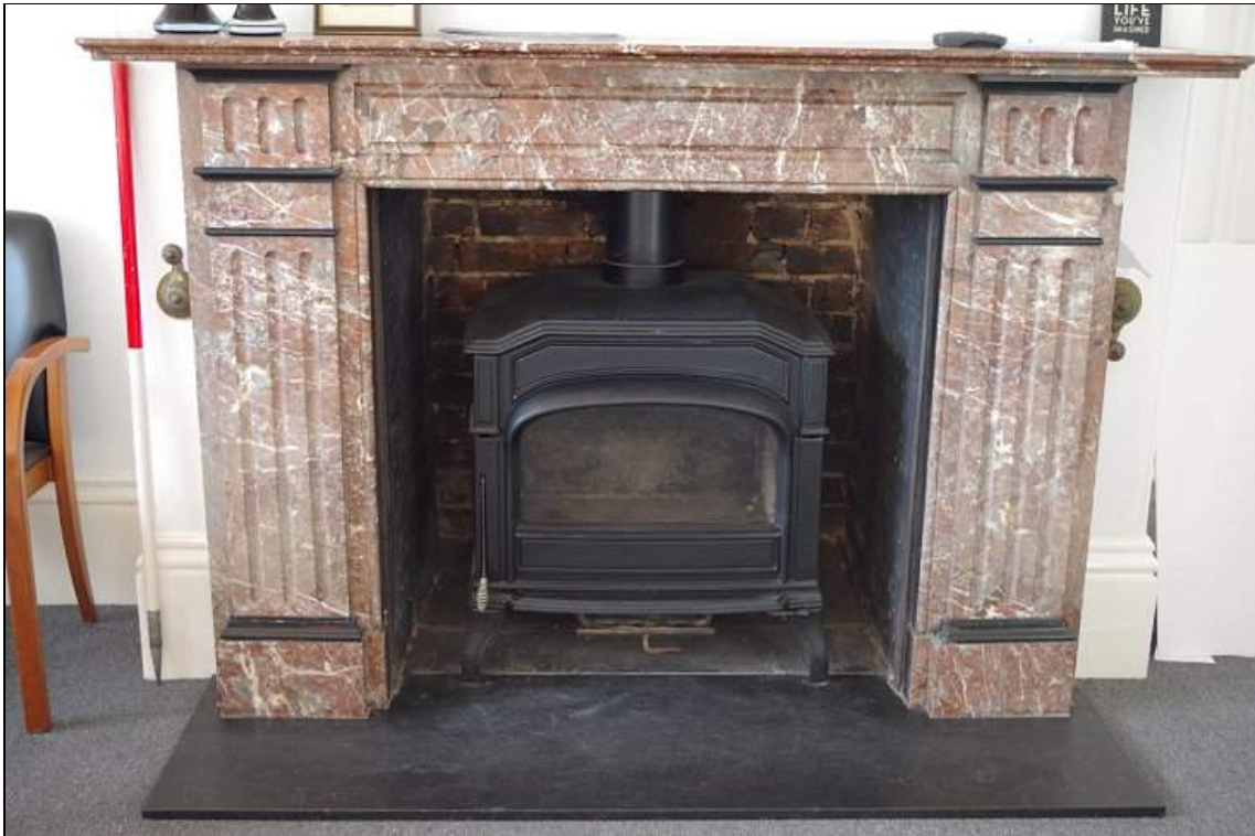
Photo 37. Victorian fireplace in SW reception room of Main Range & servant bell pulls.
