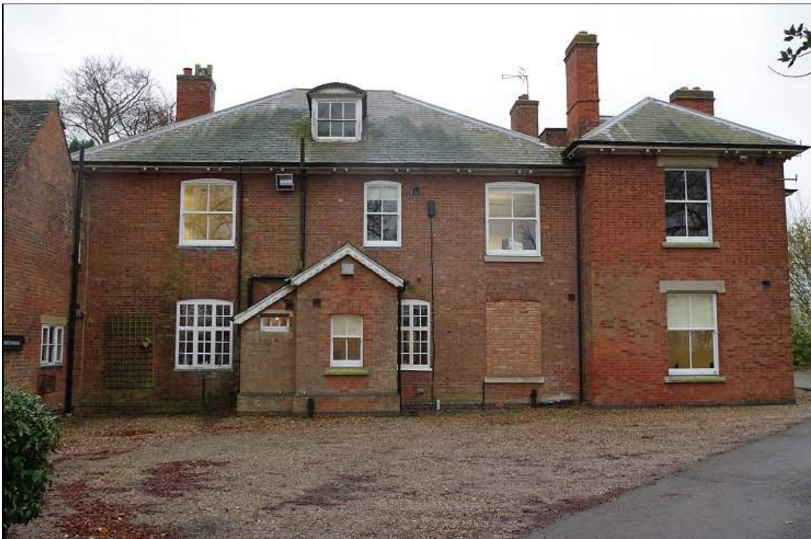
Photo 4. General view of Bittesby House from the N ( Main Range & West Range to right ).
