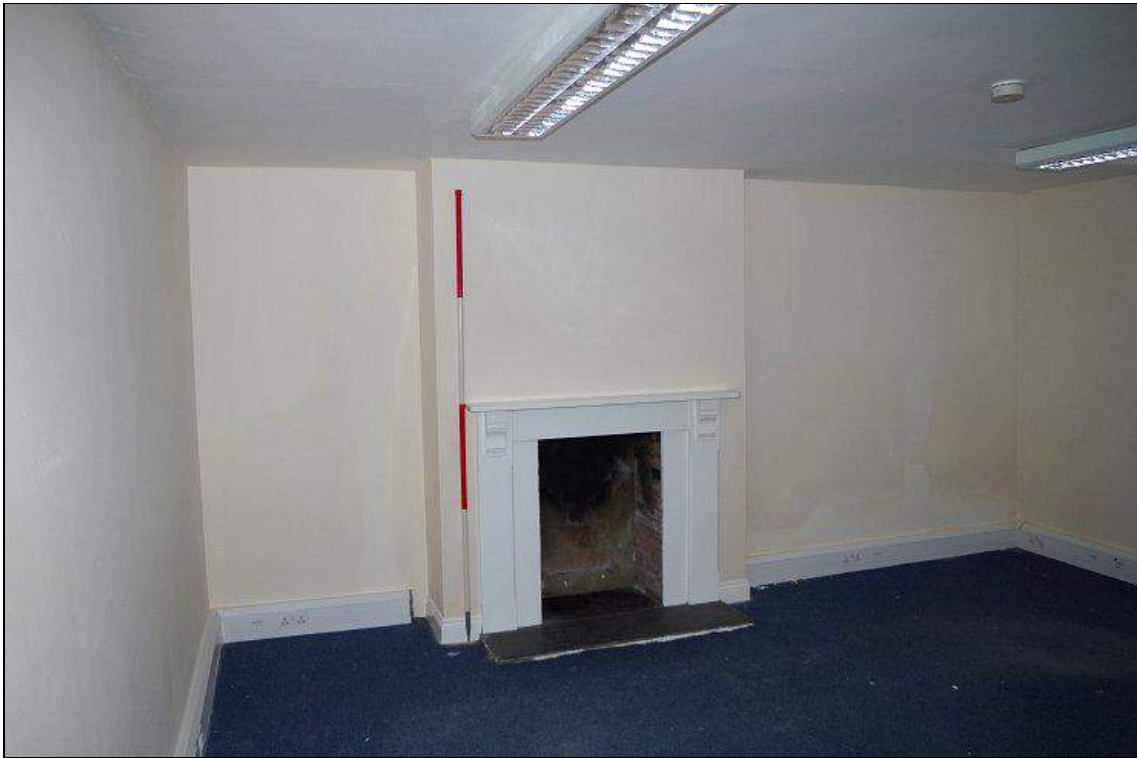
Photo 11. Ground floor E room of East Range , looking SE.
