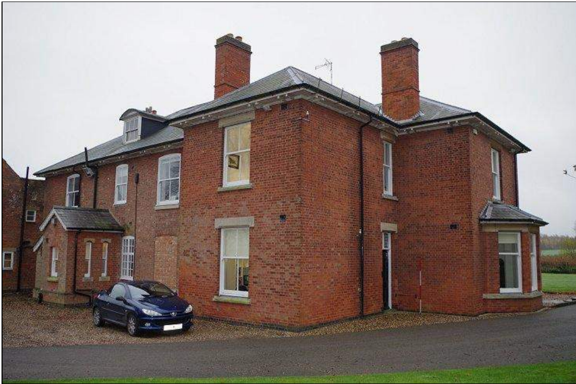
Photo 65. The West Range looking SW.
