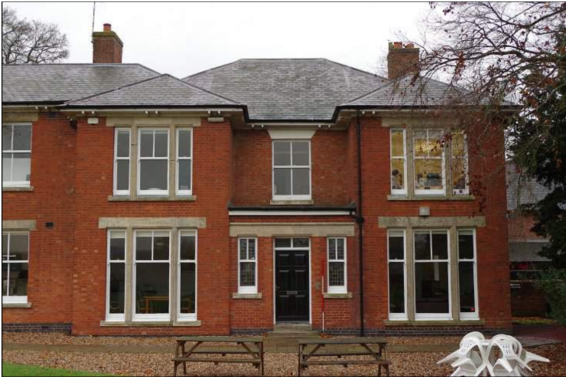
Photo 27. South Front of Main Range as rebuilt in the later 19 th century, looking N.
