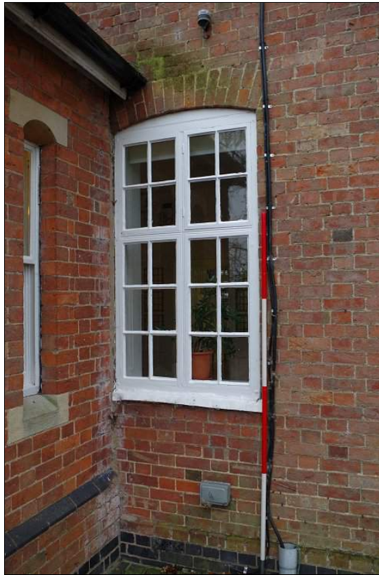
Photo 29. Early window in N elevation of Main Range , looking S.
