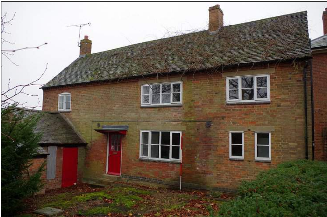
Photo 8. North elevation of the East Range , looking SSE.
