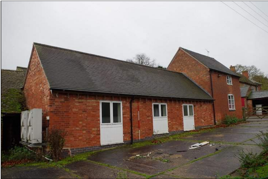
Photo 85. North front of former Cow House recently converted for office use, looking SW.
