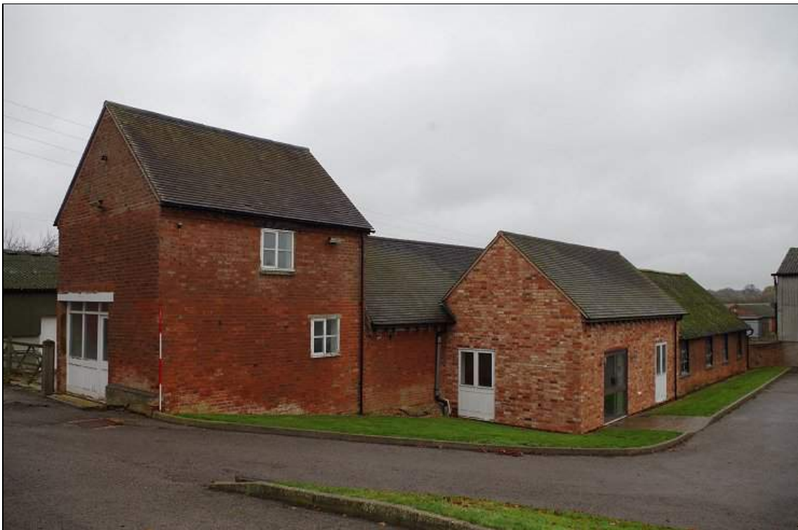
Photo 82. Former agricultural buildings on S side of yard NE of Bittesby House, looking NE.
