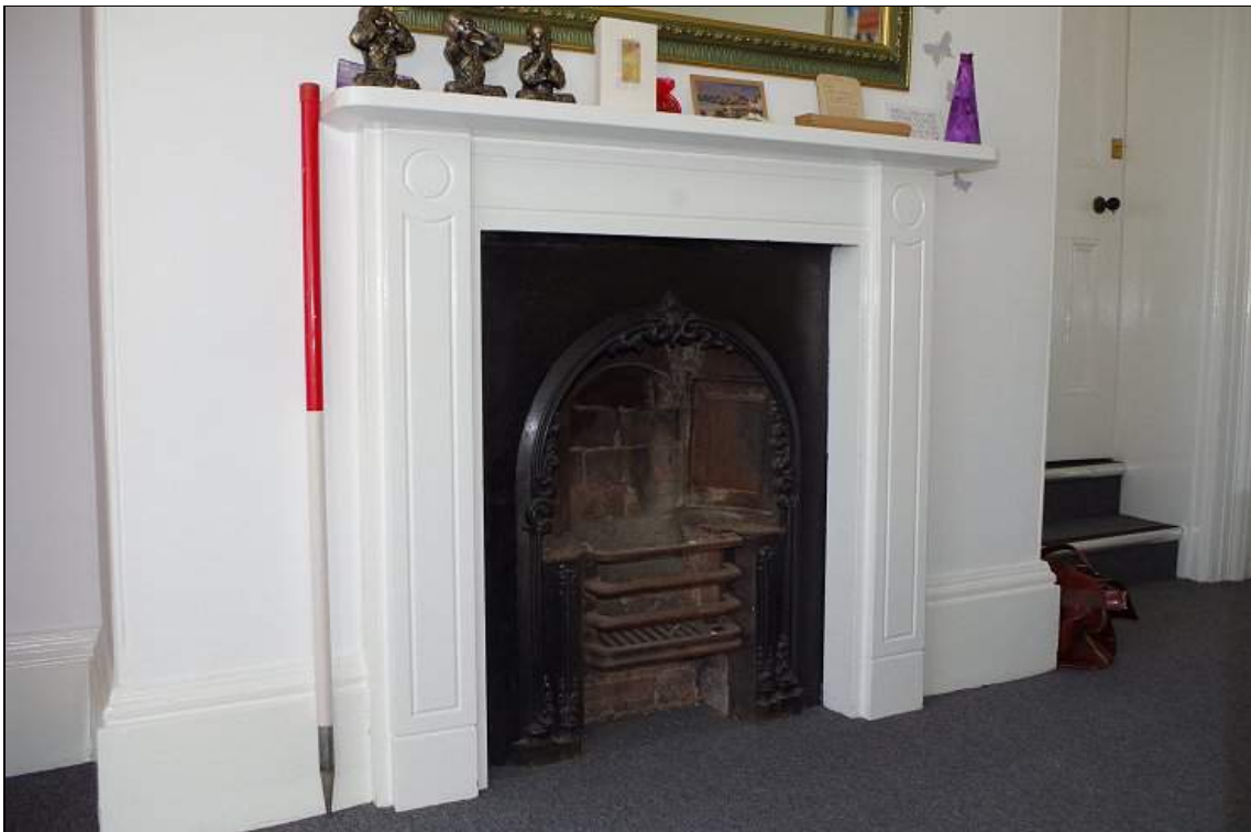
Photo 48. Fireplace in SW bedroom with stone/slate surround and arch-headed insert.
