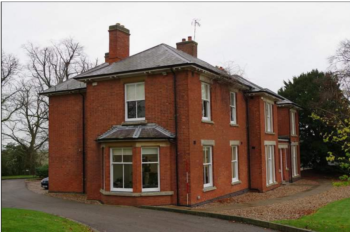
Photo 2. General view of Bittesby House from the SW.
