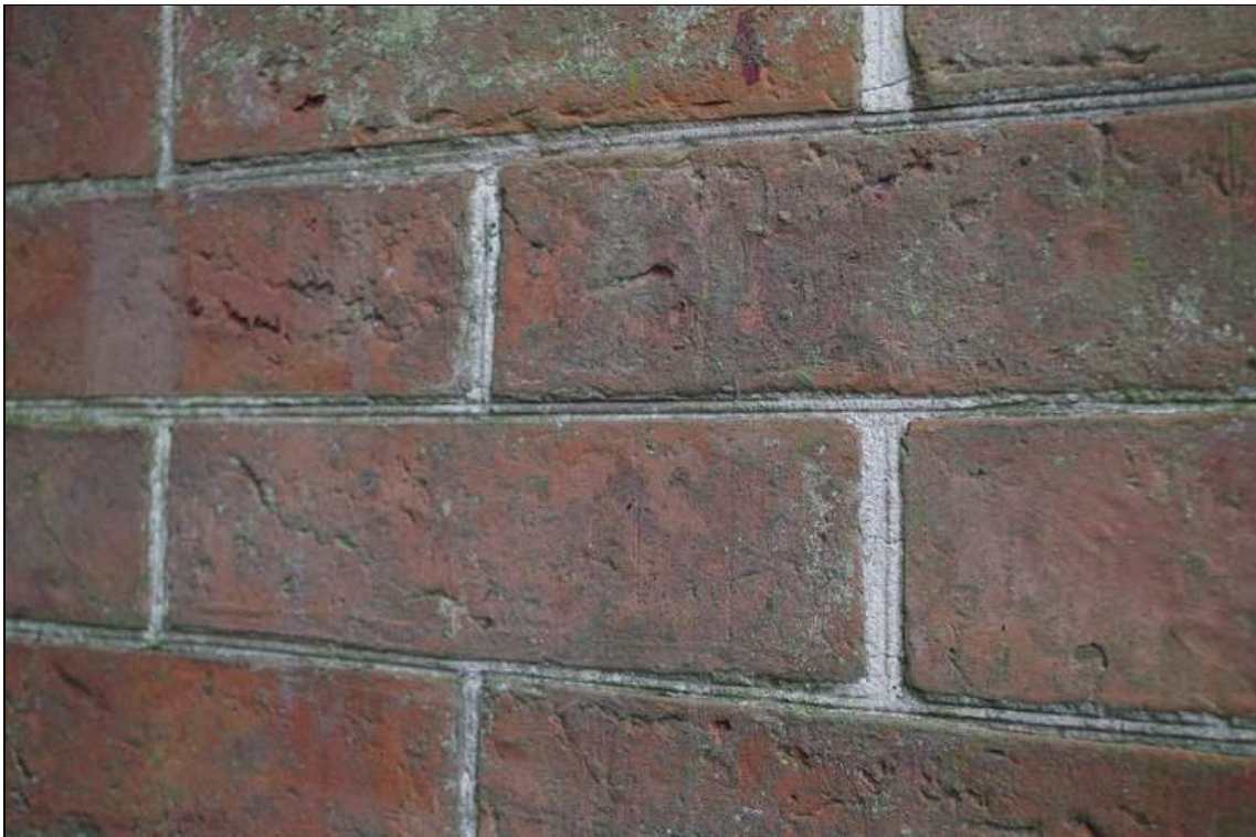
Photo 62. Detail of beaded mortar joints to brickwork of South Front .
