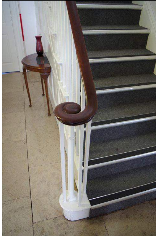
Photo 33. Detail of staircase newel, curtail step and handrail within Main Range .
