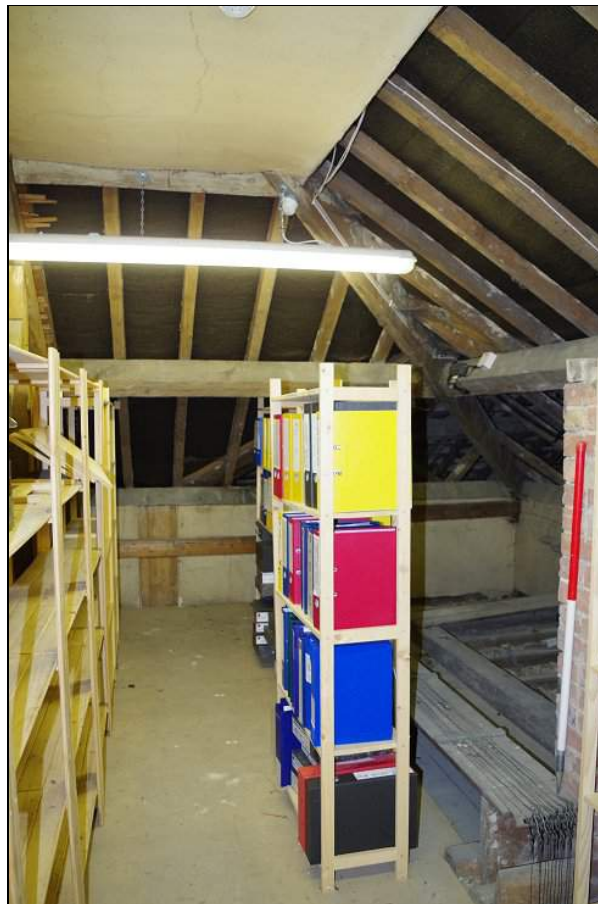
Photo 56. West attic room within Main Range , looking SW.
