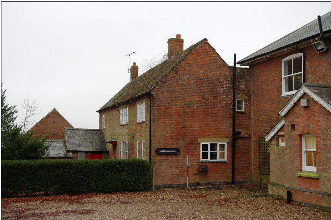
Photo 10. W elevation of East Range , looking WSW.
