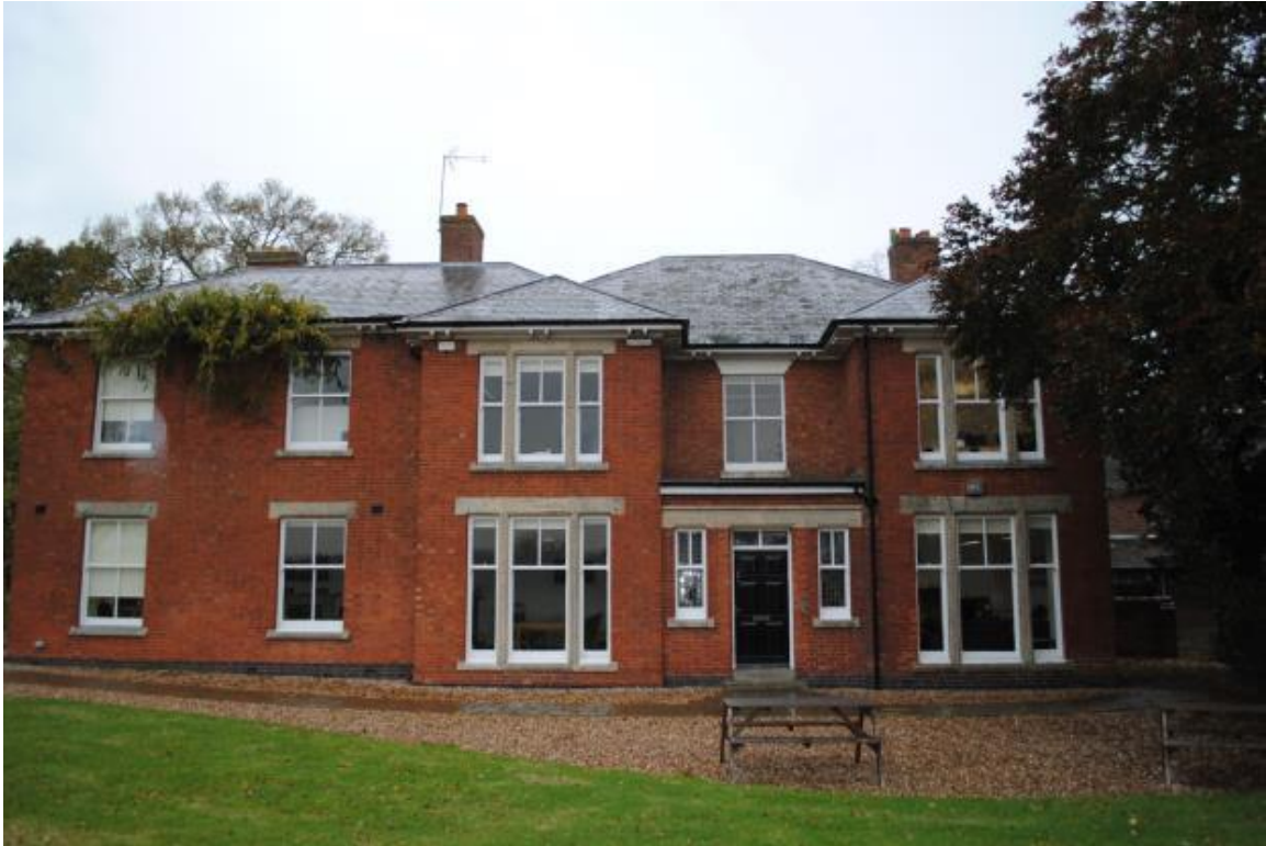
Plate 8: South elevation of Bittesby House
