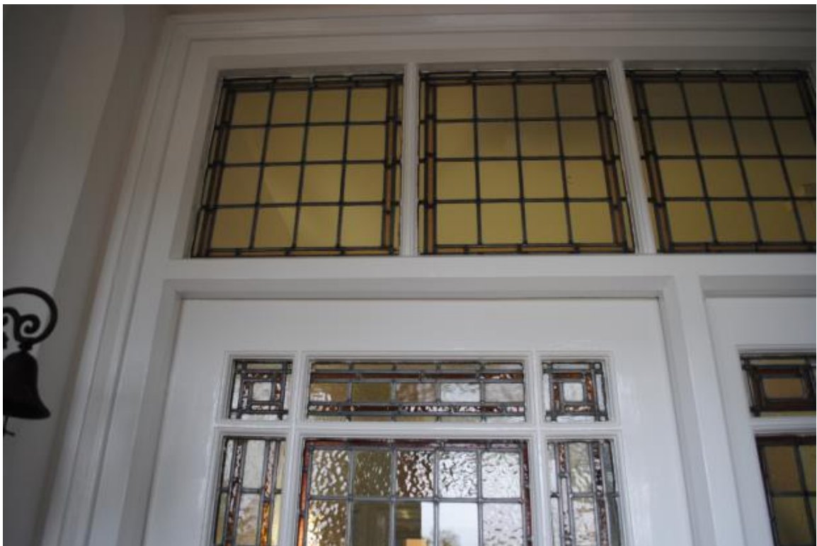
Plate 13: Internal door detail, Bittesby House
