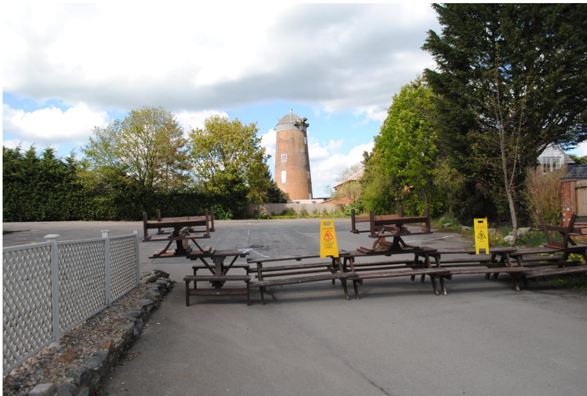
Plate 3: Ullesthorpe Mill, Ullesthorpe. As viewed looking north over Country Chequers Inn carpark, Main Street
