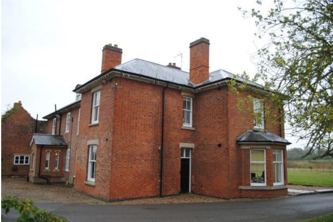
Plate 10: South-west and north-west elevation of Bittesby House
