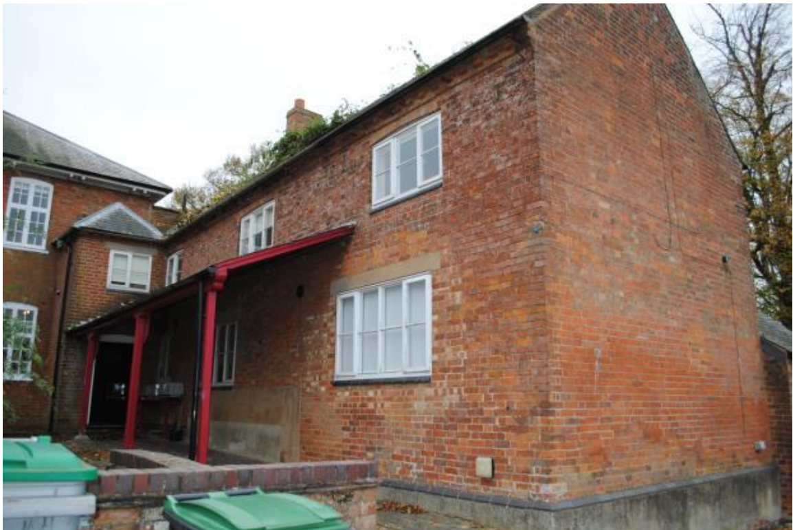
Plate 7: South-east elevation of Bittesby House
