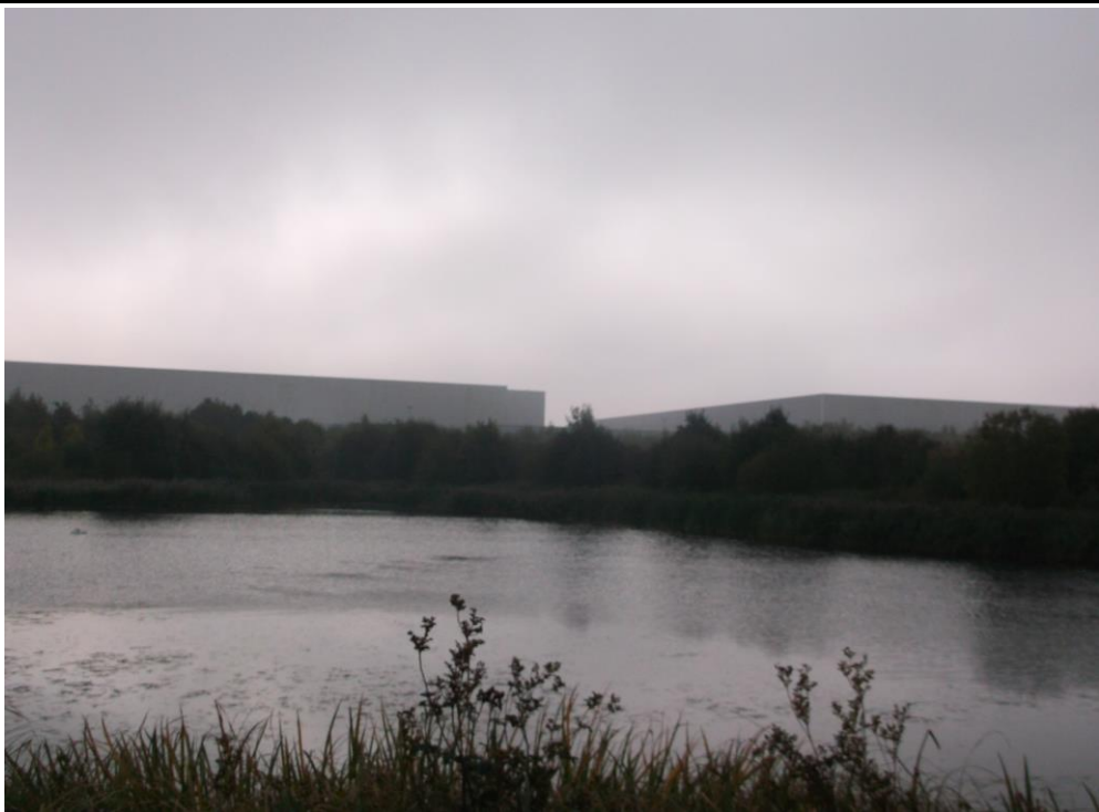
Photograph 18 – Drainage lagoon associated with the existing Magna Park.
