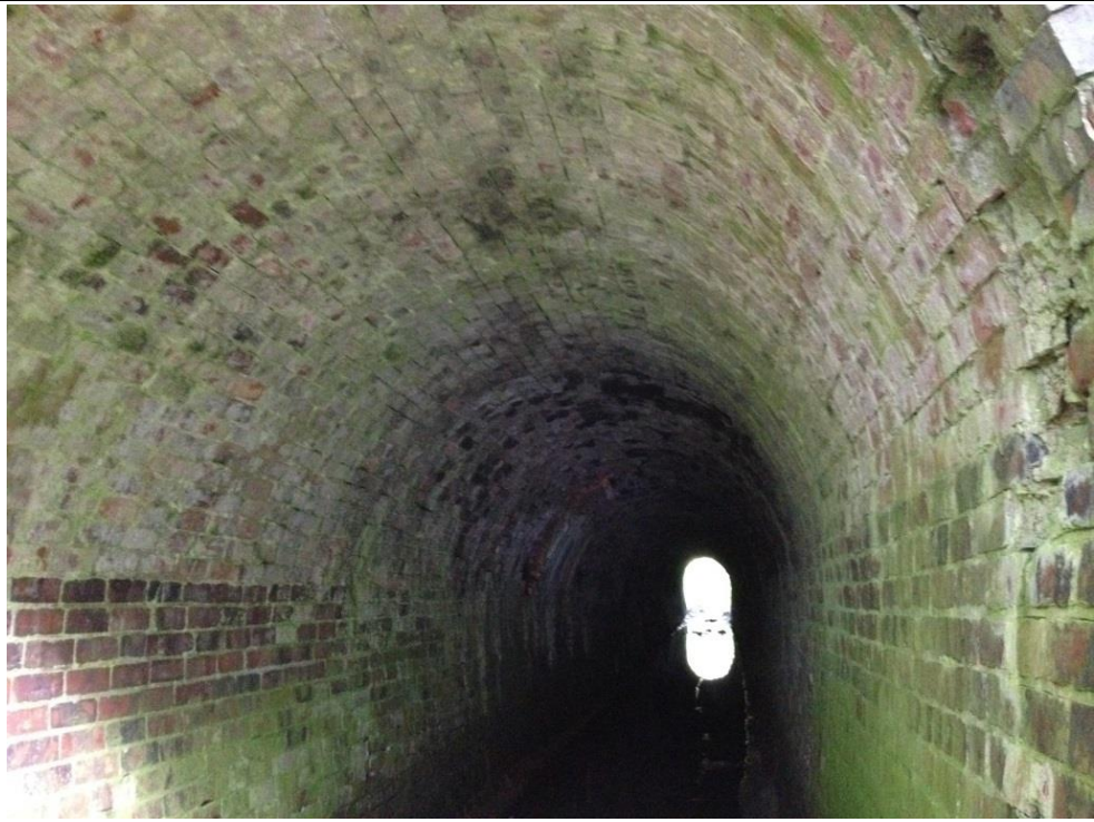
Photograph 7 – Tunnel for brook crossing beneath the railway embankment.
