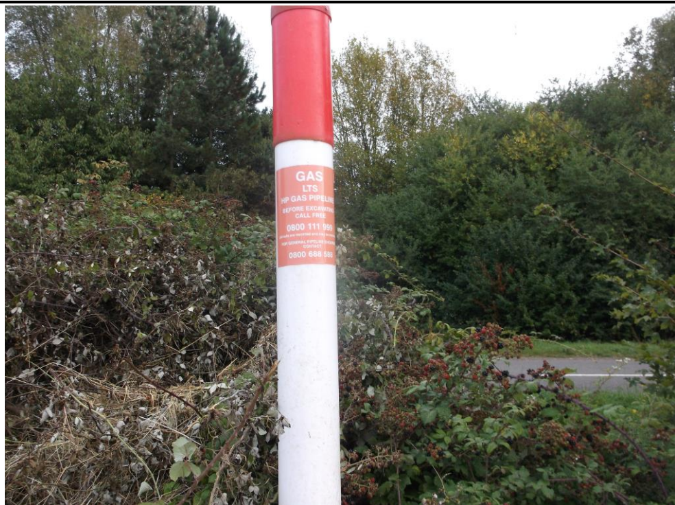
Photograph 12 – High pressure gas pipeline within Site boundary, alongside Mere Lane.
