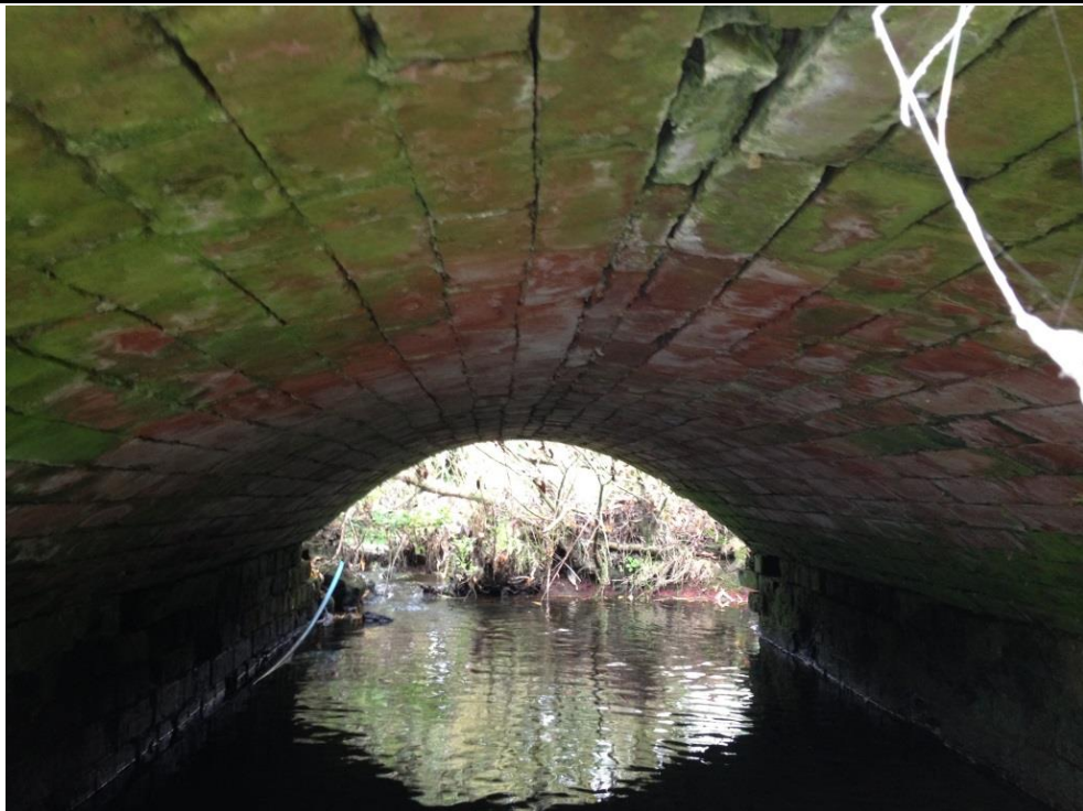
Photograph 8 – Second tunnel for brook crossing beneath the railway embankment.
