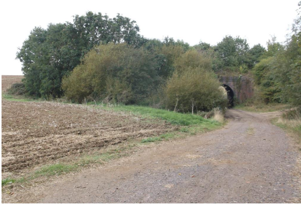
Photograph 9 – Vehicular access tunnel through railway embankment.
