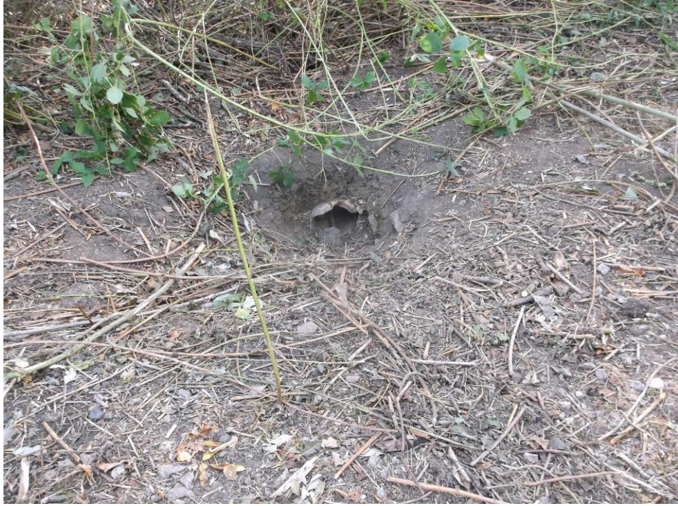
Photograph 13 – Collapsed drainage pipe near lagoon.
