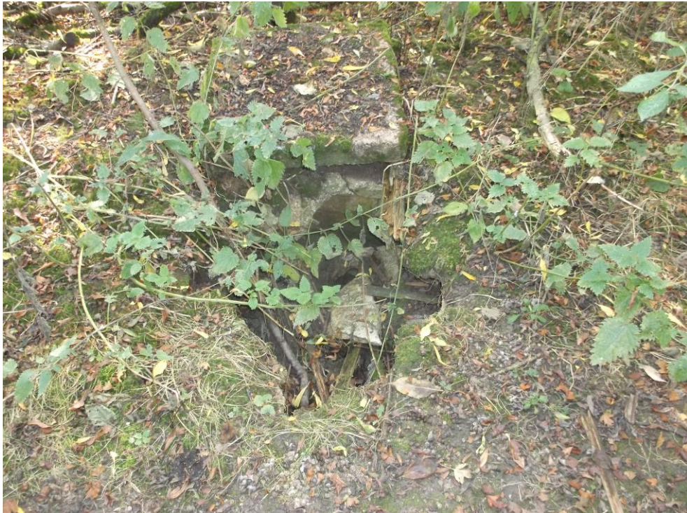
Photograph 14 – Second collapsed manhole near lagoon.
