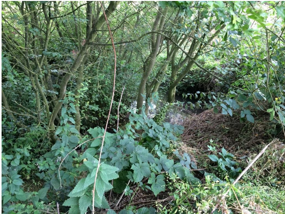
Photograph 5 – A section of Drain 5 along the woodland edge
