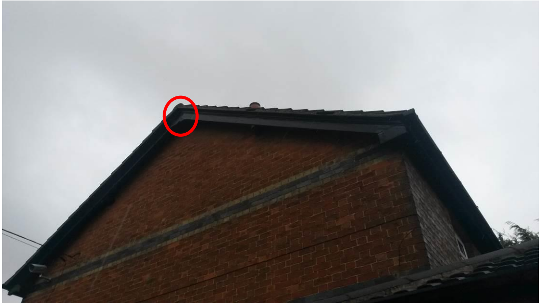
Photograph 1 – Eastern gable end of Lodge Cottage, roost location within red circle
