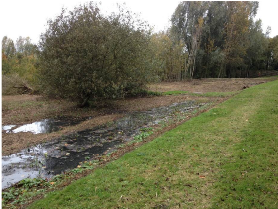
Photograph 8 – Reed bed undergoing renovation / improvement works
