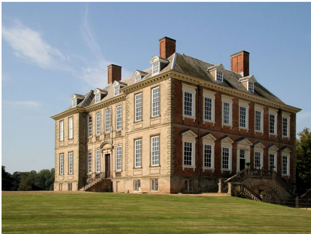
Figure 4.13: Grade I listed building: Stanford Hall, south east of Lutterworth
