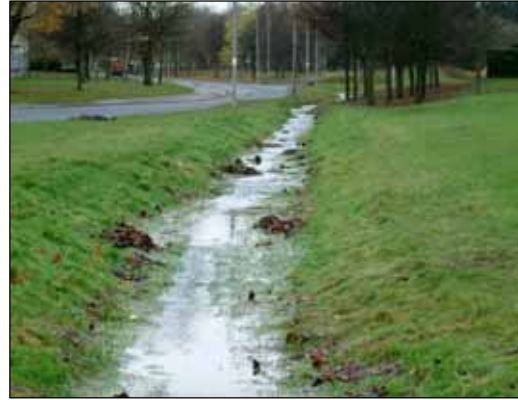
Figure 18: A swale in operation (Source: SUDSnet v )
