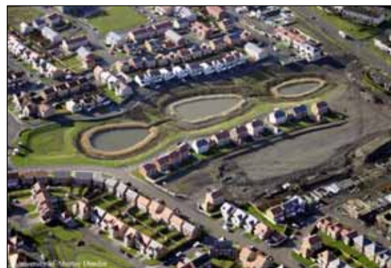
Figure 22 Retention ponds (Source: SUDSnetv)
