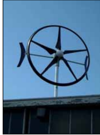
Figure 4: 1.5 kW building mounted wind turbine (2 m diameter)
