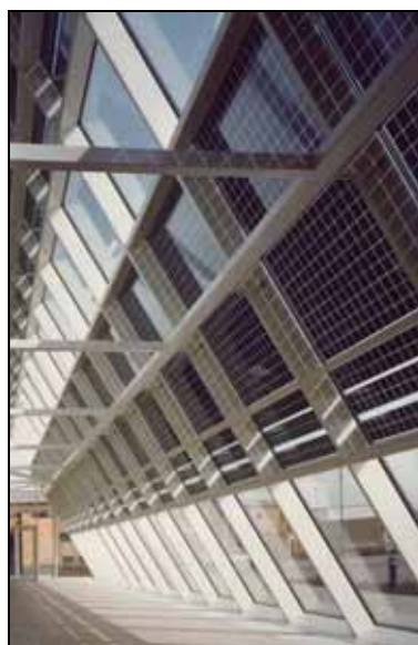
Figure 28: Internal appearance of the 73 kWp array
