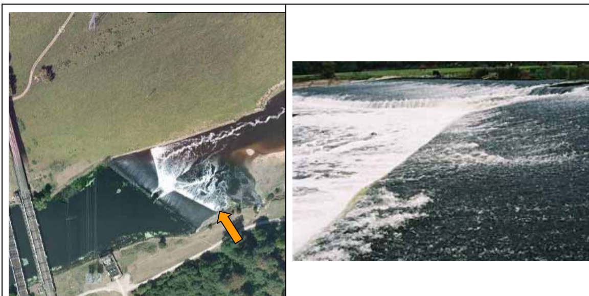
Figure 21: Ratcliffe Power Station Weir – River Trent
