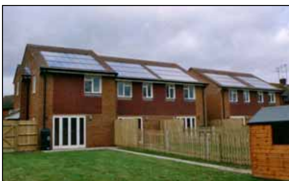
Figure 25: 5 x 1.75 kWp roof integrated PV arrays
