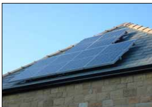
Figure 26: 0.75 kWp non-integrated PV array
