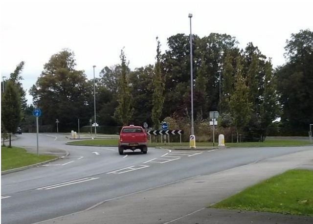
The new A6 roundabout at junction with Wistow Road
