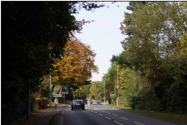
The 'new' route of the A6
