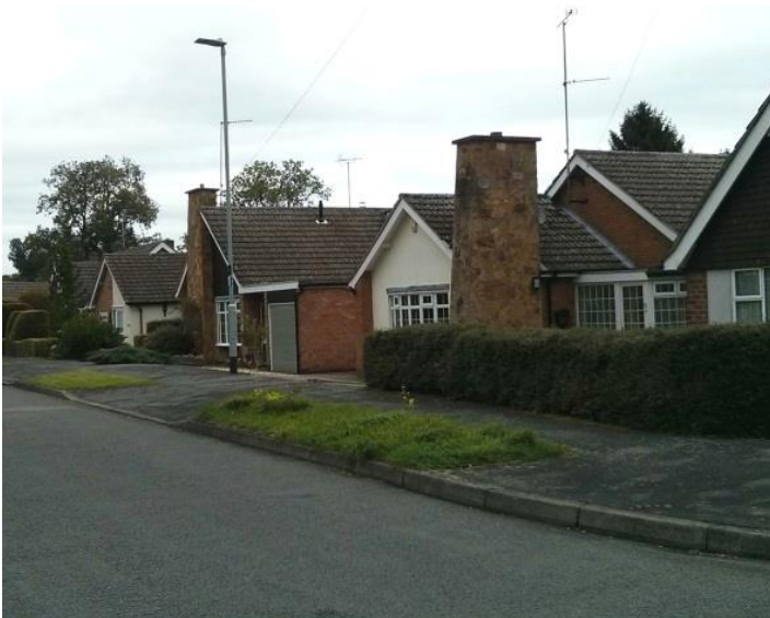
Marsh Avenue, off Langton Road, has many bungalows
