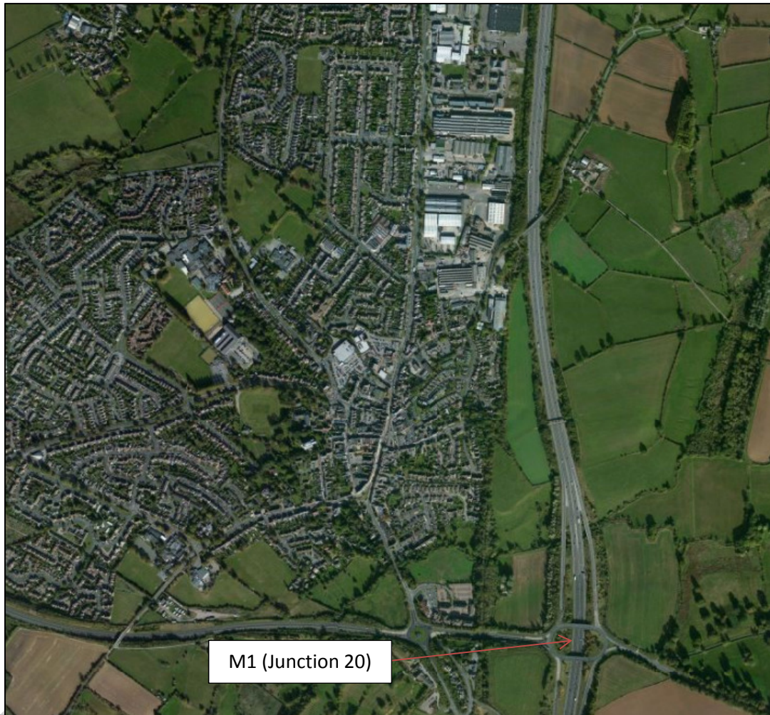
Figure 6.2: Location of (M1 Junction 20)
