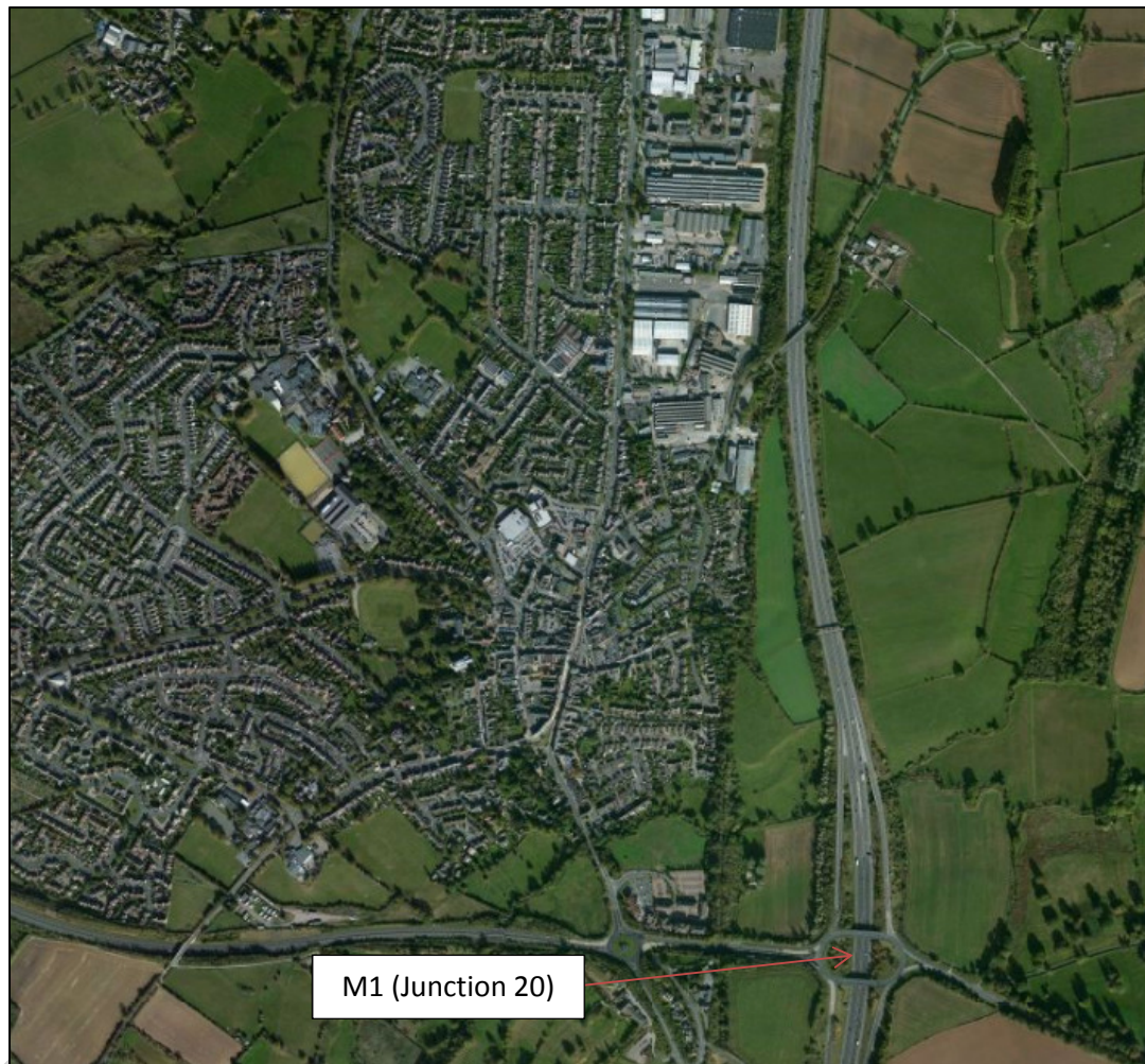
Figure 6.2: Location of (M1 Junction 20)
