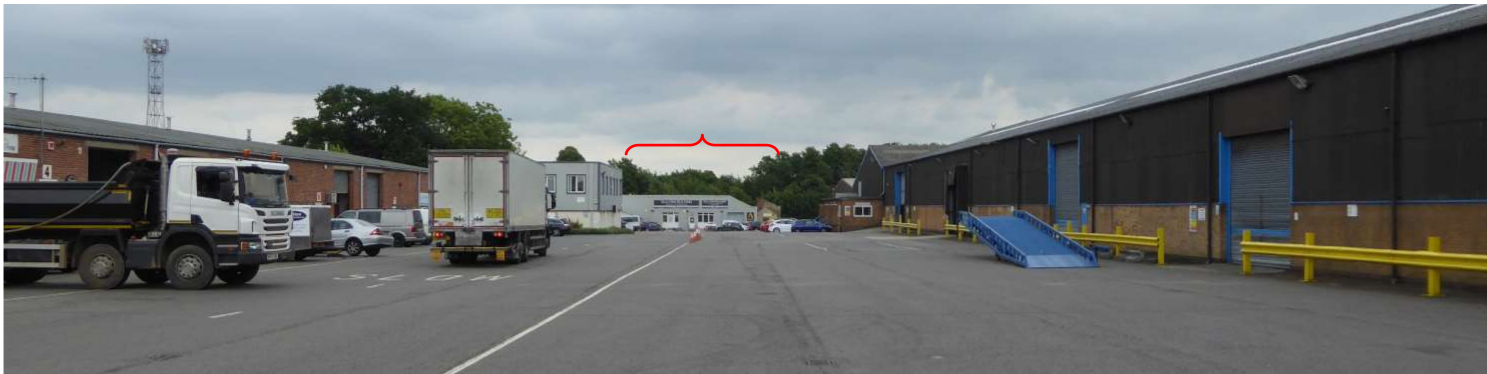
Plate 34: A long view east towards the Ladywood Works along Leicester Road.
