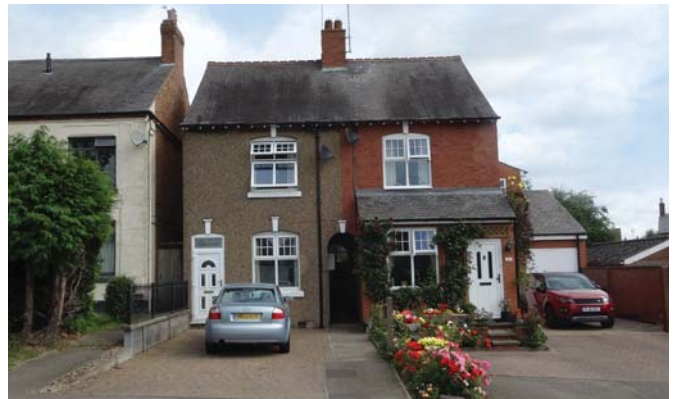
Semi-detached homes on Kilby Road
