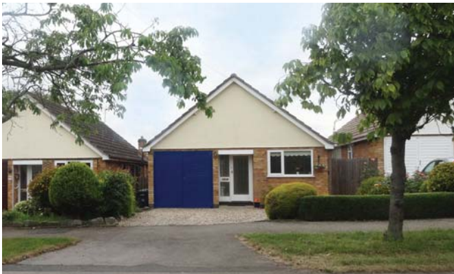
Bungalow situated on Leicester Road
