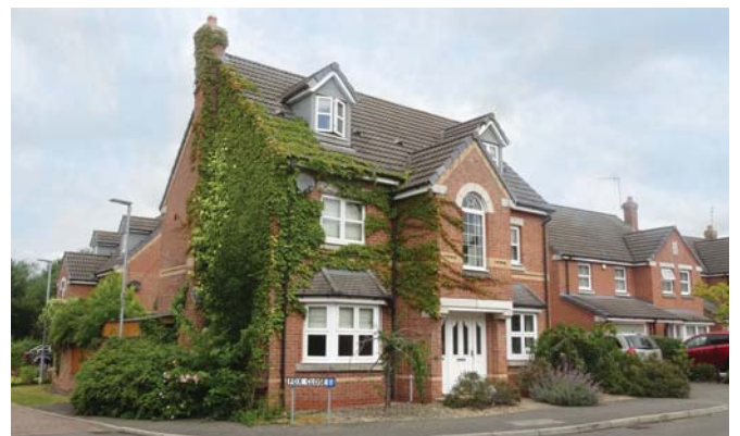
Two-and-a-half storey dwelling on Badcock Way
