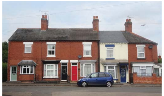
Terraced block on Gladstone Street
