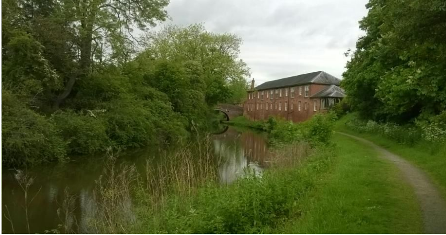
Figure 2. View from the towpath looking north.
