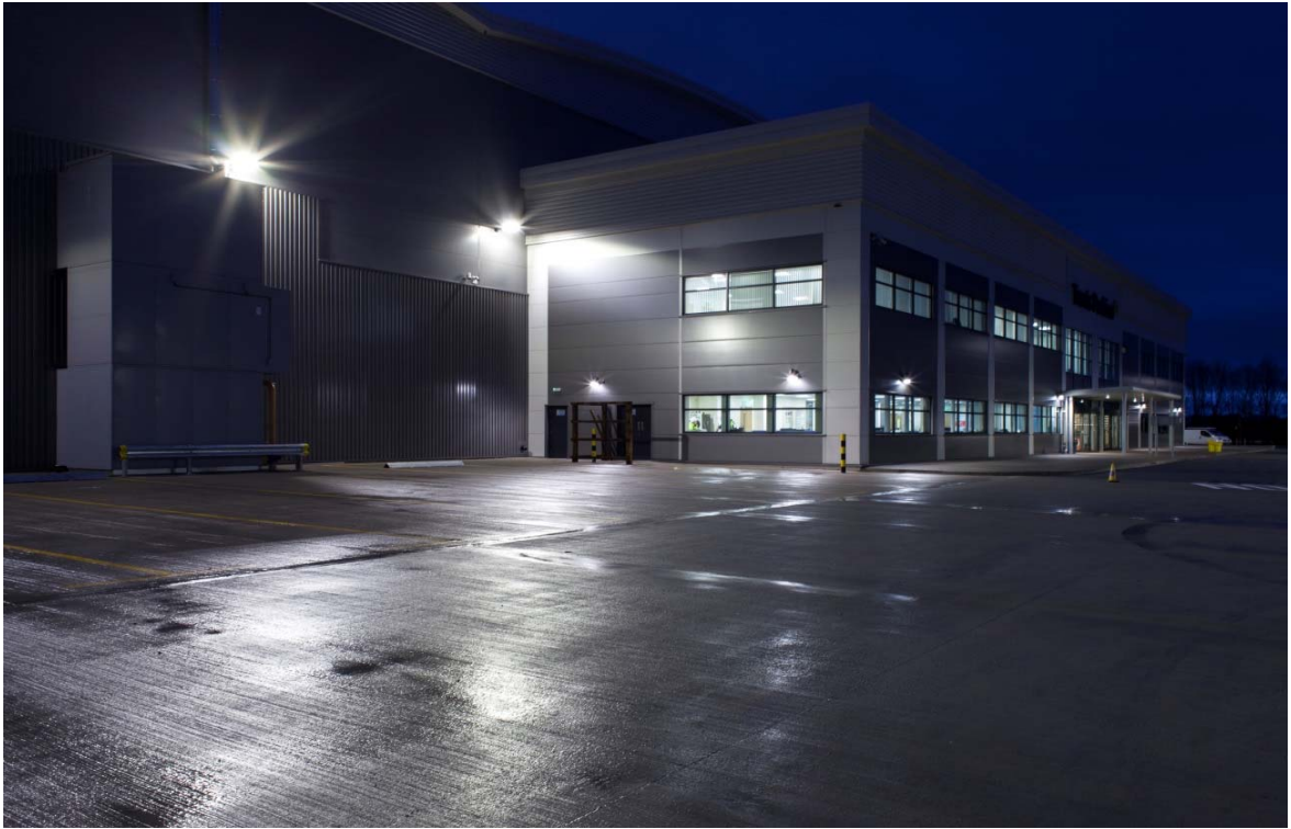
Building illumination greatly reduced (Low intensity light source with 0.2% upward light)
