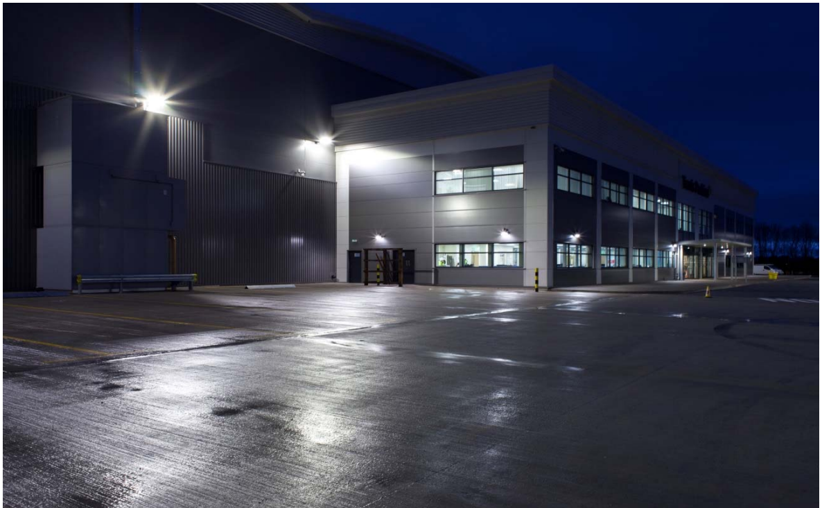
Upper half of building in darkness due to low mounting height and reduced reflectance
