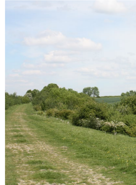
Figure 13b The existing railway embankment
