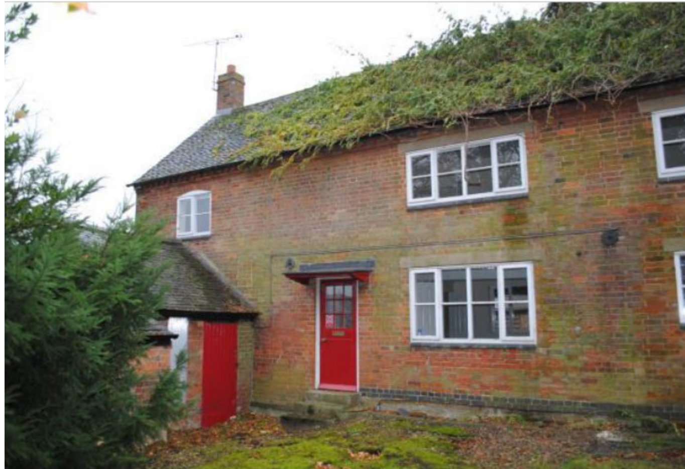
Figure 24: North elevation of the Eastern Range of Bittesby House
