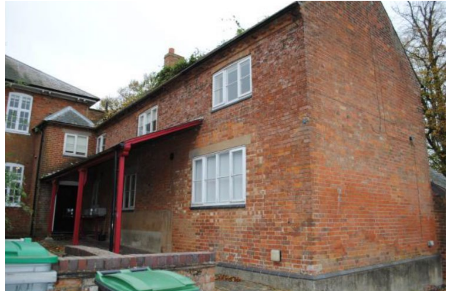
Figure 25: South east elevation of the Eastern Range of Bittesby House
