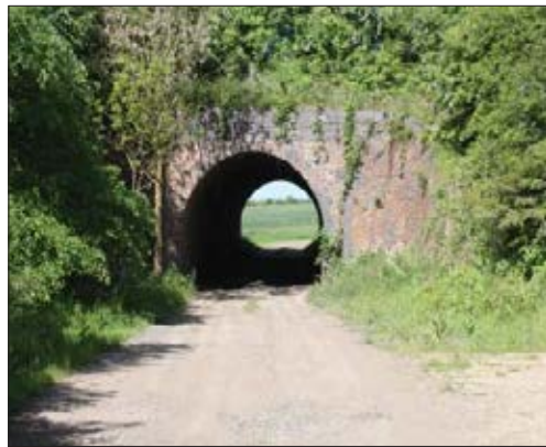
1. Heritage features - former disused railway to Ullesthorpe.
