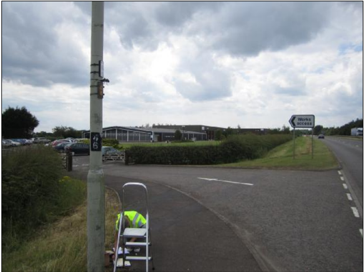
Figure G4.2: Monitoring Location 2 – A4303, On Lamppost, Near Entrance to TT Electronics
