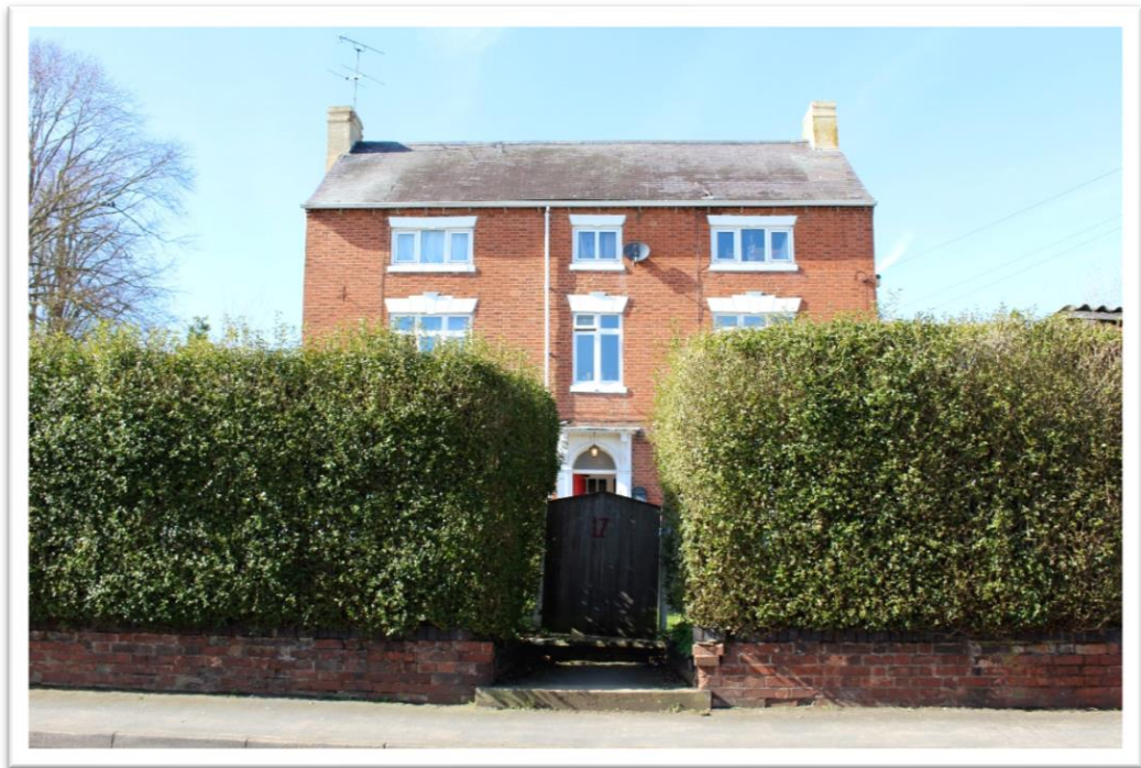
FIGURE 2: THE MANOR HOUSE
