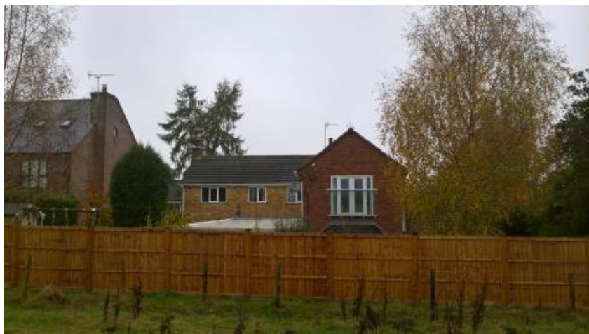
Figure 12 - Photographs showing the rear elevations of some of the dwellings on the east side of Little Lunnon, taken from the site
