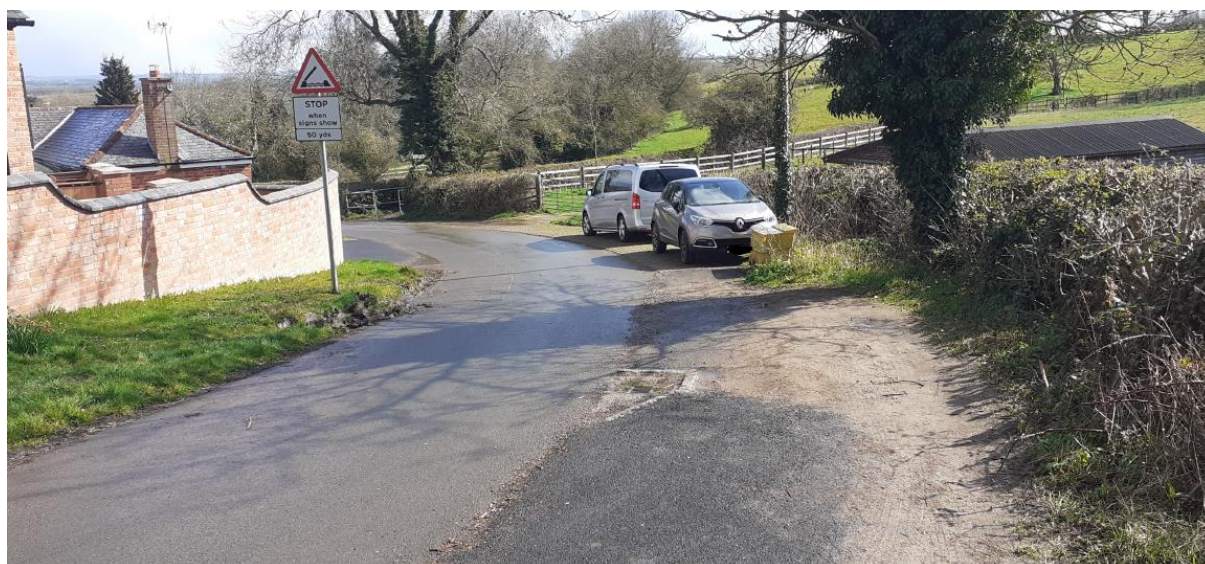
Figure 3: View looking east along Swingbridge Street towards PRow A22
