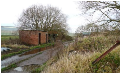
Fig 08 - Existing Agricultural Building for Demolition
