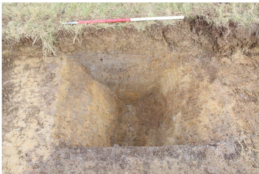
Plate 7: An elevated view of ditch [1204] and recut [1207] showing the straight, steeply sloping sides and pointed base (Section 12.1). The recut is located below the red part of the scale. See also Figure 5 (1m scale; looking east).
