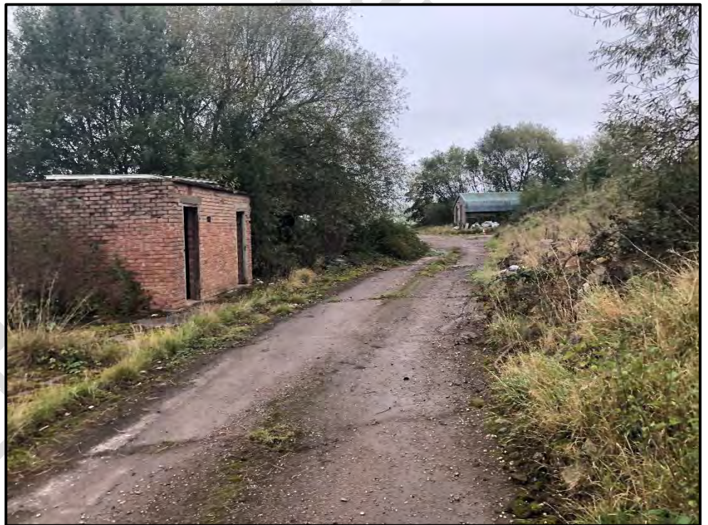
Plate 3: Brick building, Nissen Hut obscured by vegetation and modern storage structure and former runway surface, looking north
