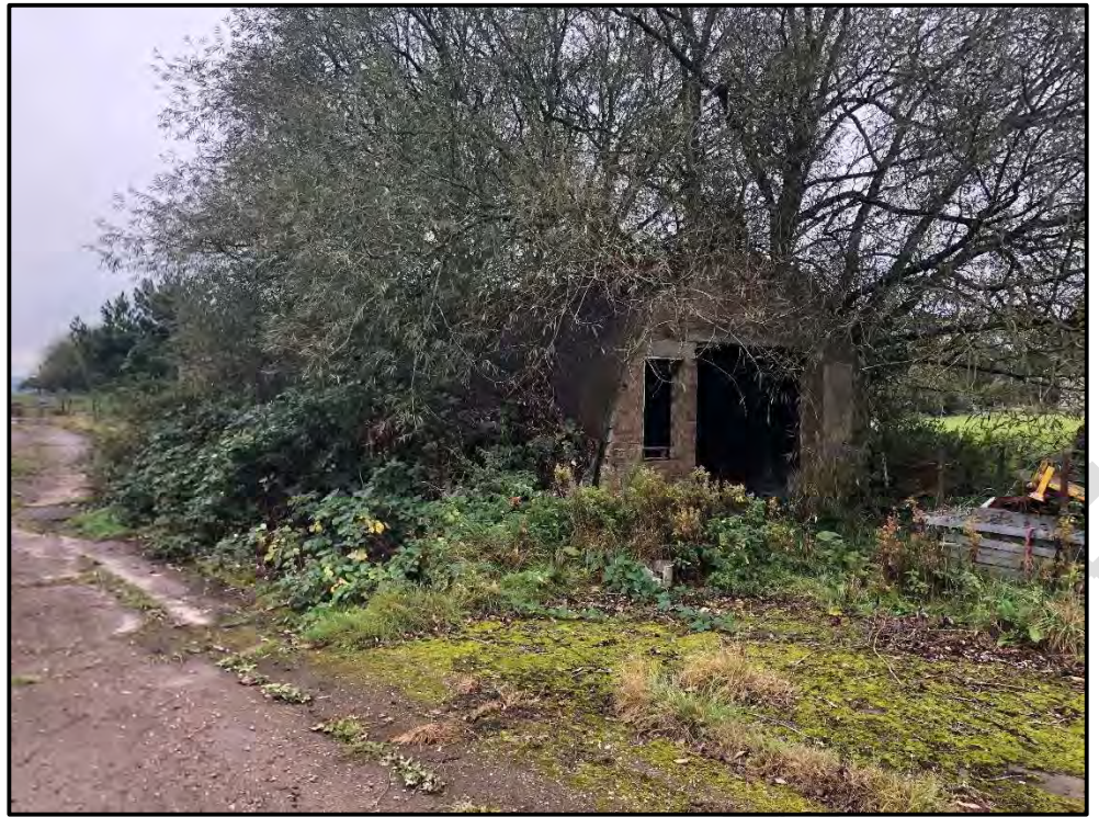
Plate 2: Northern and eastern elevation of Nissen Hut at the north east of the study site, looking south
