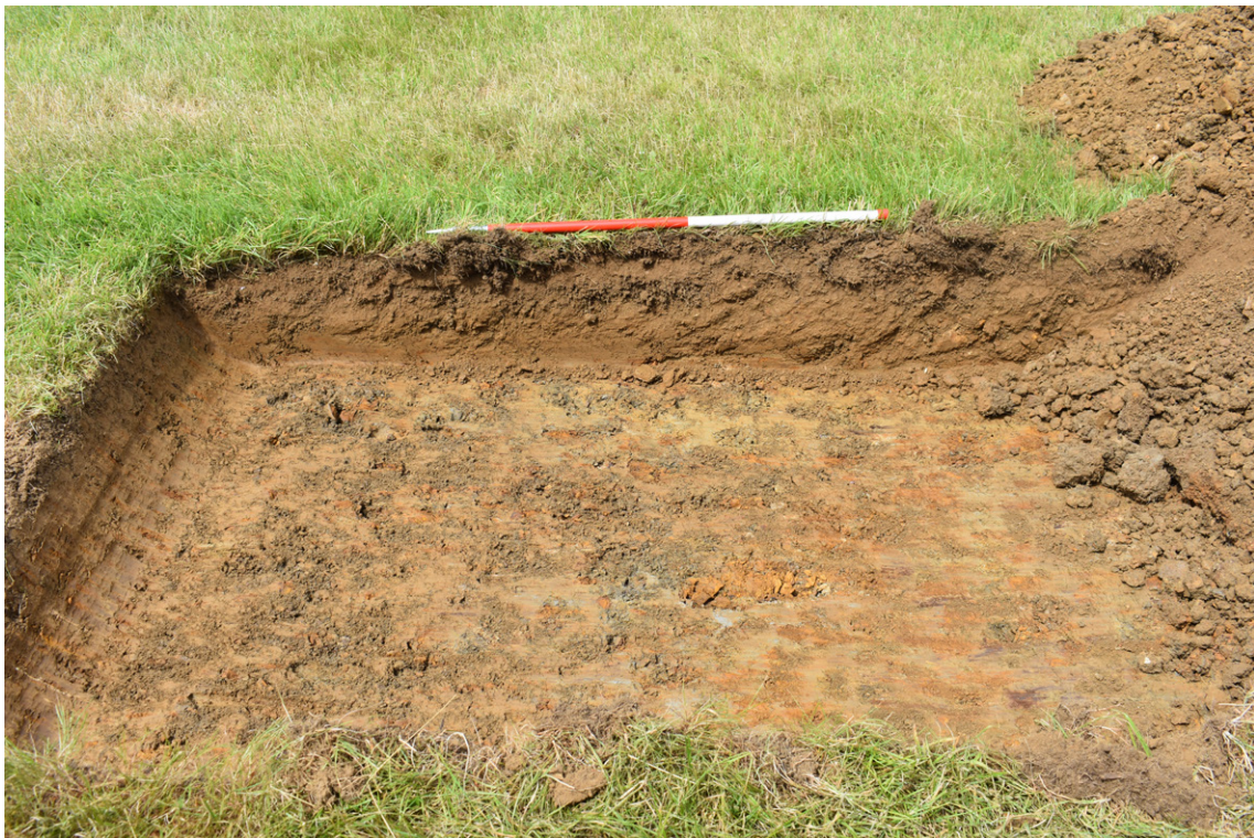
Fig. 3.4: North facing shot of CBR Test Pit 108
