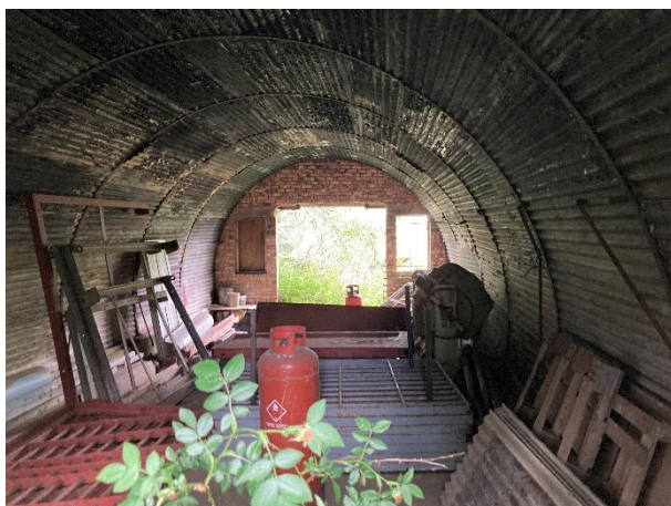
Plate 1- Interior of B1.
