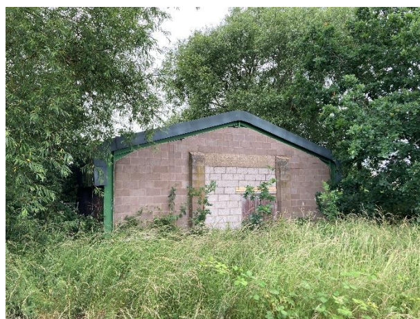
Plate 4 – B2 rear (east) elevation.
