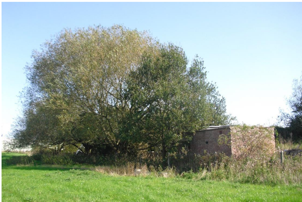
Photo 8. Small brick building with low bat roosting potential (TN10)
