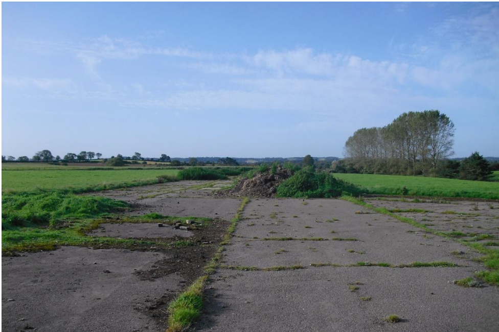
Photo 14. A view southwest along the long strip of hardstanding with vegetated manure piles to the south of the existing prison (TN3)
