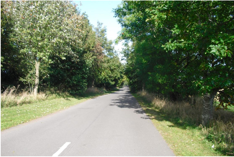
Photo 9. A view northeast along Welland Avenue, bordered by lines of scattered trees
