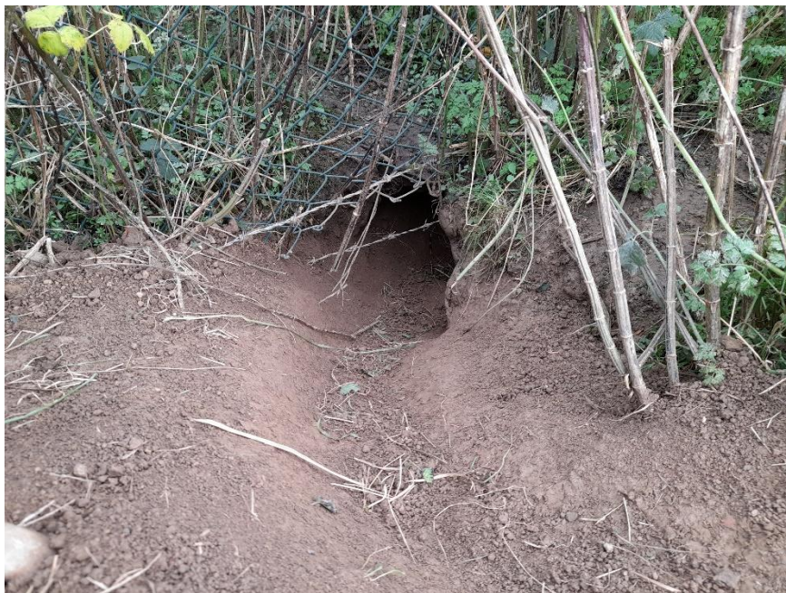
Photo 2. An S1 entrance which undermines the farm track
