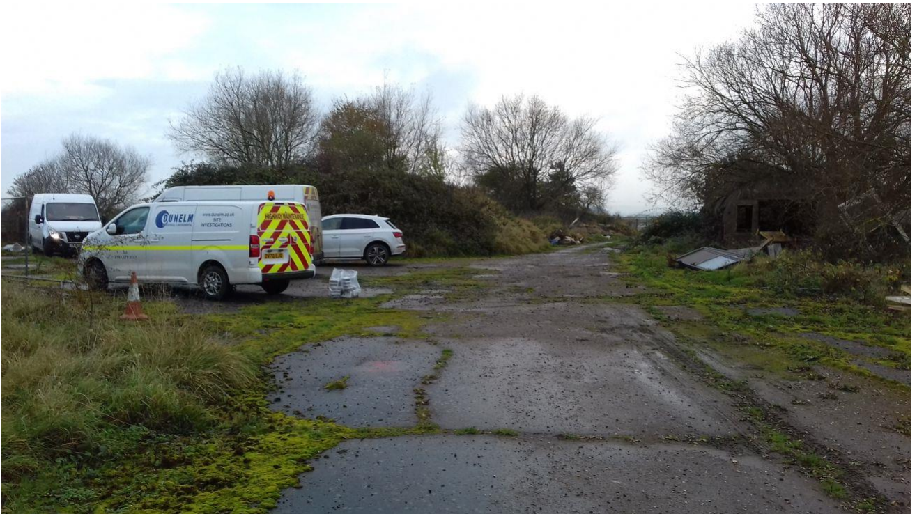
4 Rough hardstanding area in the north of the site
