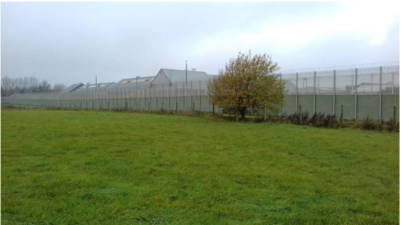
2 General view of site looking towards existing prison
