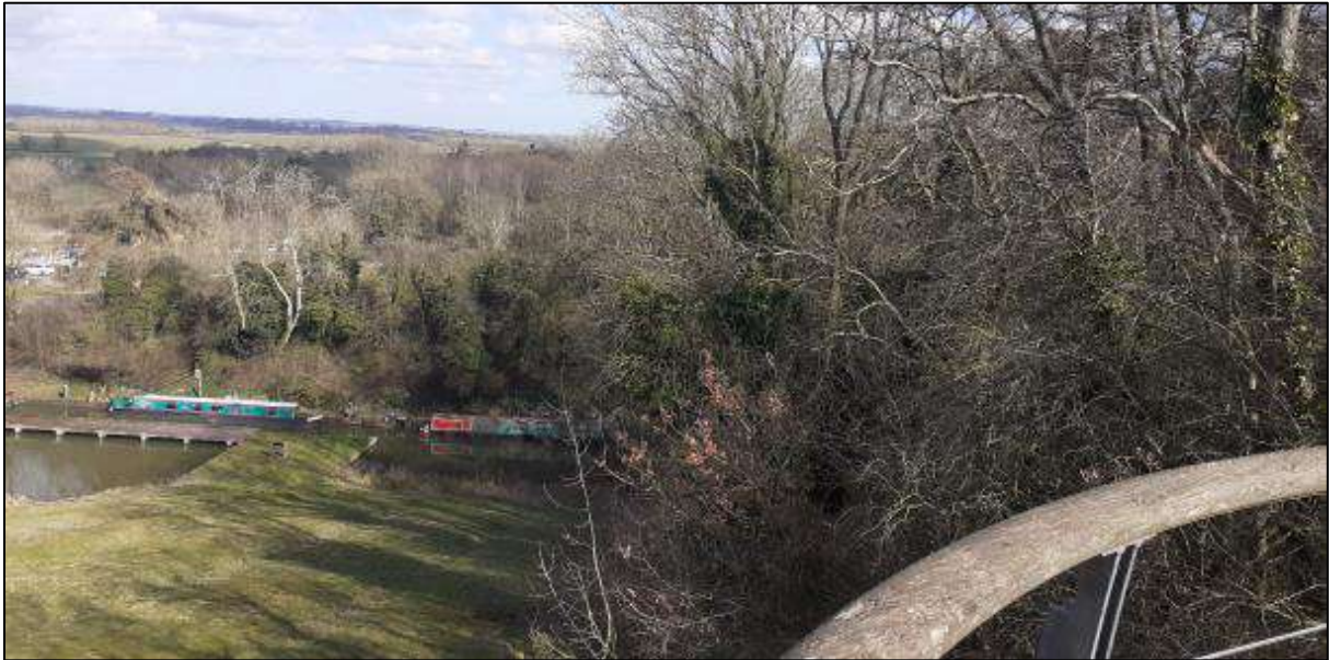
Figure 30: View of Foxton Inclined Plane from viewing platform
