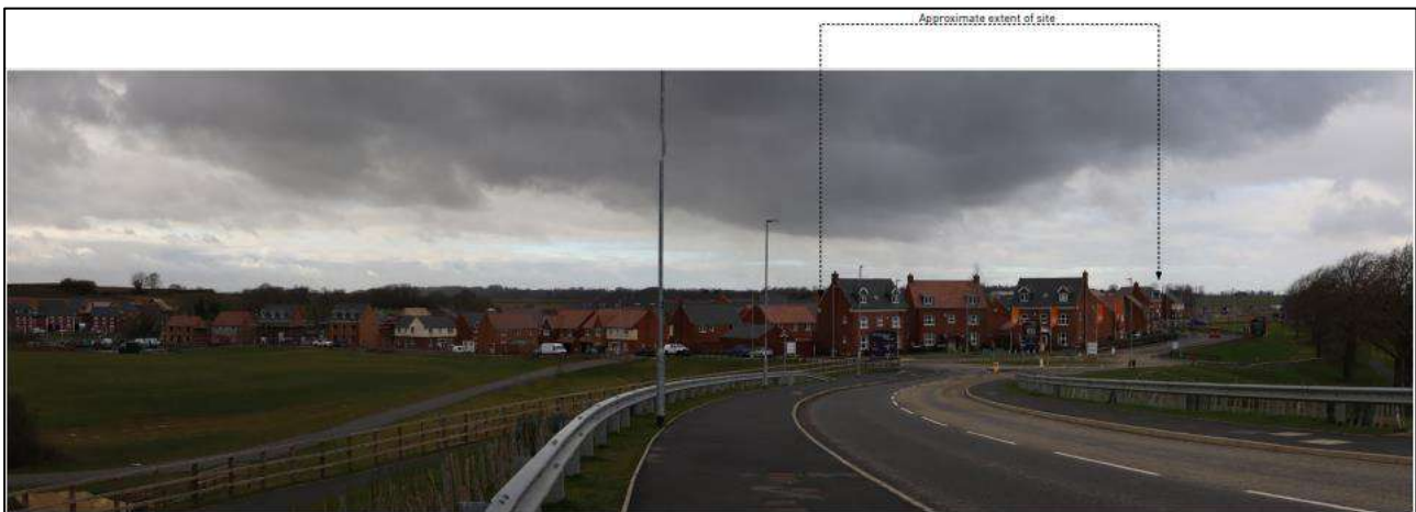
Figure 61: View of site from Peter Callis Way above canal towpath (Viewpoint 10)
