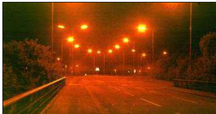
Figure 66: Example of High pressure Sodium lamps
