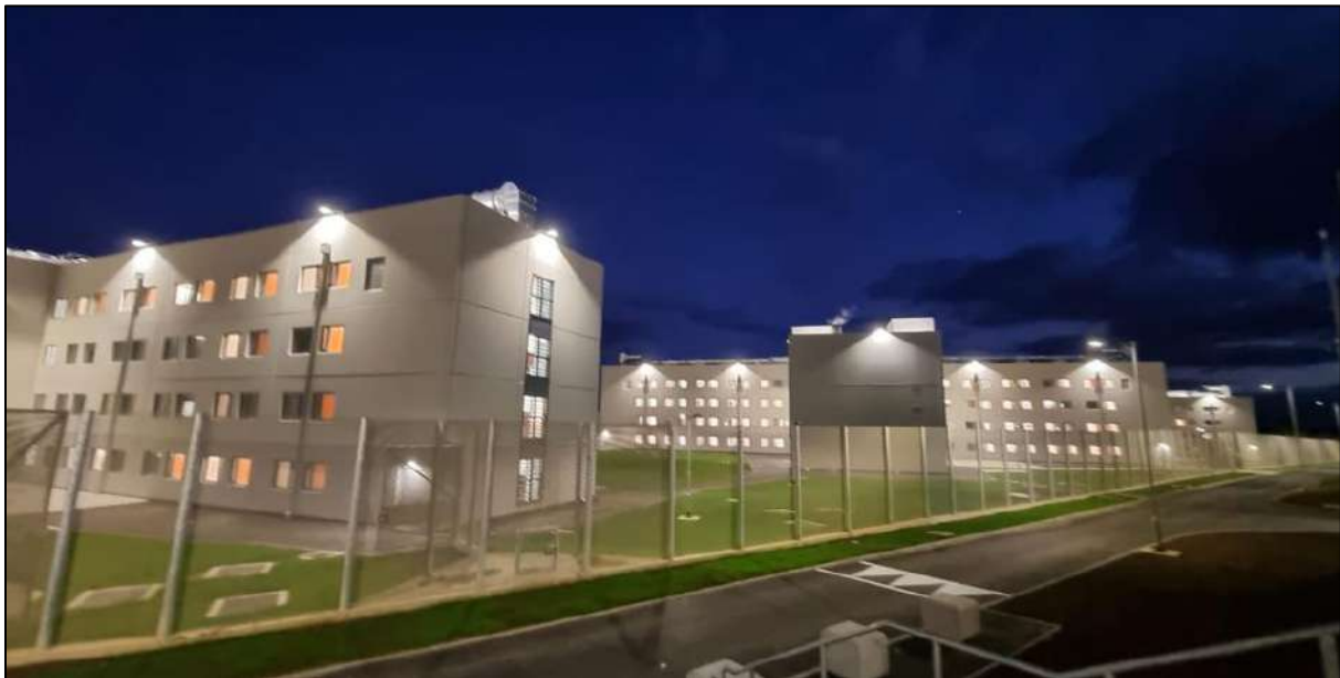
Figure 67: Example of LED Lighting on a Prison complex
