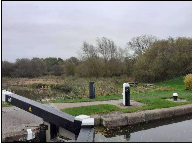
Figure 28: View across Foxton Locks towards the application site from the Top Lock
