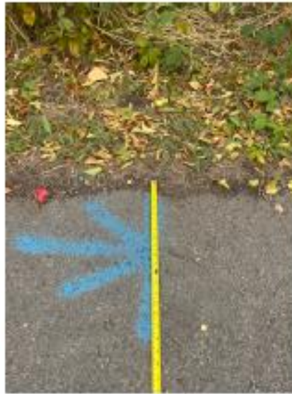
Picture 6. The tape is positioned at the edge of the road
