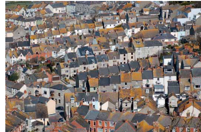
Figure 2.2 'Townscape' means the landscape within the built-up area, including the buildings and the relationships between them
