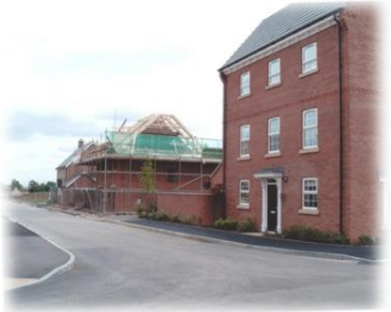
Fig. 2.4 Example of windows
