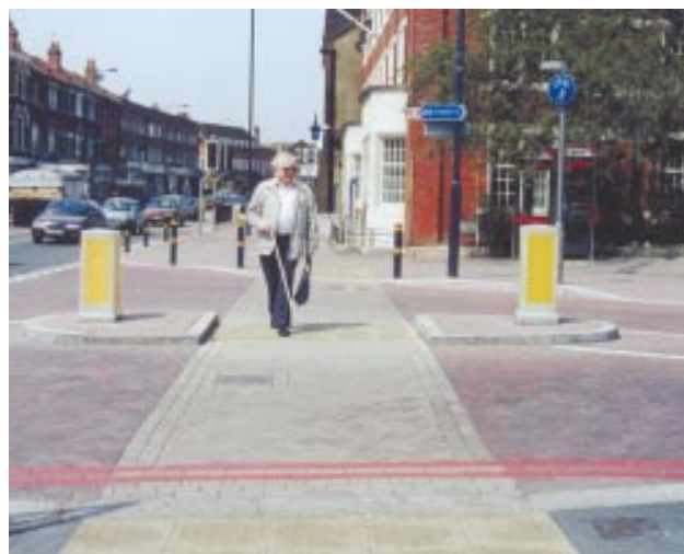
Entry treatments are common on roads joining Red Routes in London. Courtesy: TfL.
