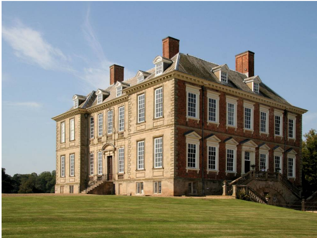
Figure 7.2: Grade I listed building: Stanford Hall, south east of Lutterworth
