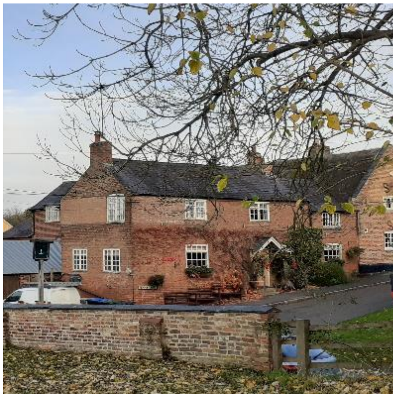
The Chandlers on the corner of Fenny Lane, viewed from The Green.
