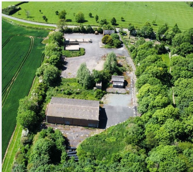
Figure 8: Former Highway Depot
