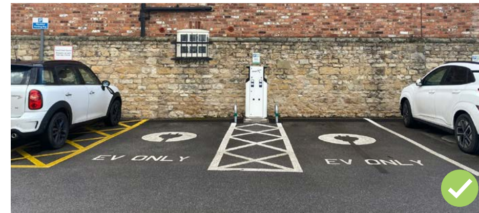
Figure 122: Example of an electric vehicle charging point provided within a parking court, serving multiple vehicles.
