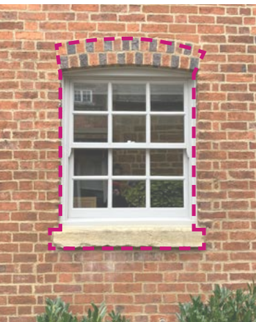
Figure 43: Sash window set within a brick facade, featuring a brick arch and stone sill.
