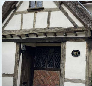
Tudor-style timber beams
