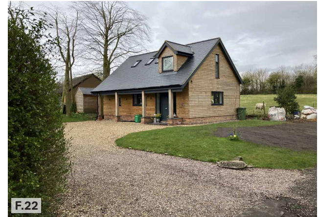
Figure 22: Example of permeable paving used on a driveway in Shearsby, coupled with grass to aid in flood management.
