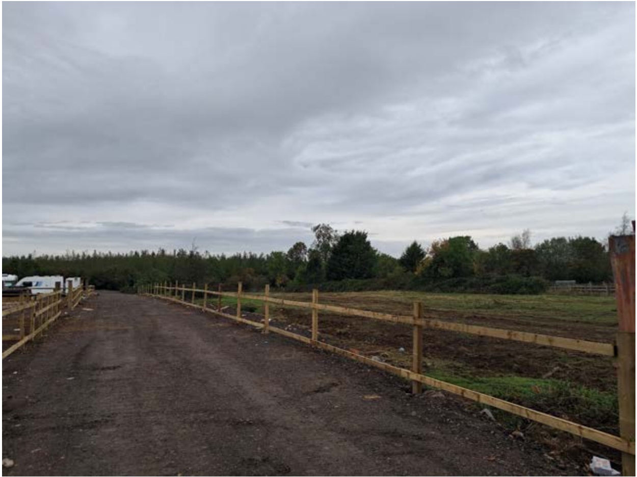
New track installed through the centre of the site to access individual pitches on the left hand side and paddock land on the right.
