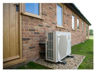
**Figure 52:** Air source heat pump unit located to the rear / side elevation of a dwelling, so to avoid its visual impact on the dwellings frontage and wider streetscape
