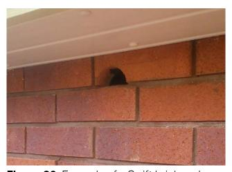
**Figure 30:** Example of a Swift brick under an eave
