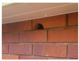
Figure 24: Example of a Swift brick under an eave
