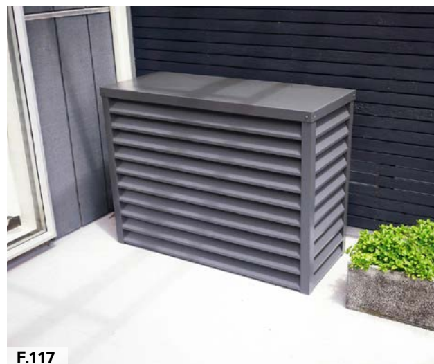
Figure 116: Air source heat pump unit.
