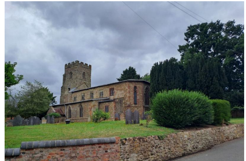
Figure 4: Swinford Churchyard: West sub-area (TEP ID: 178)
