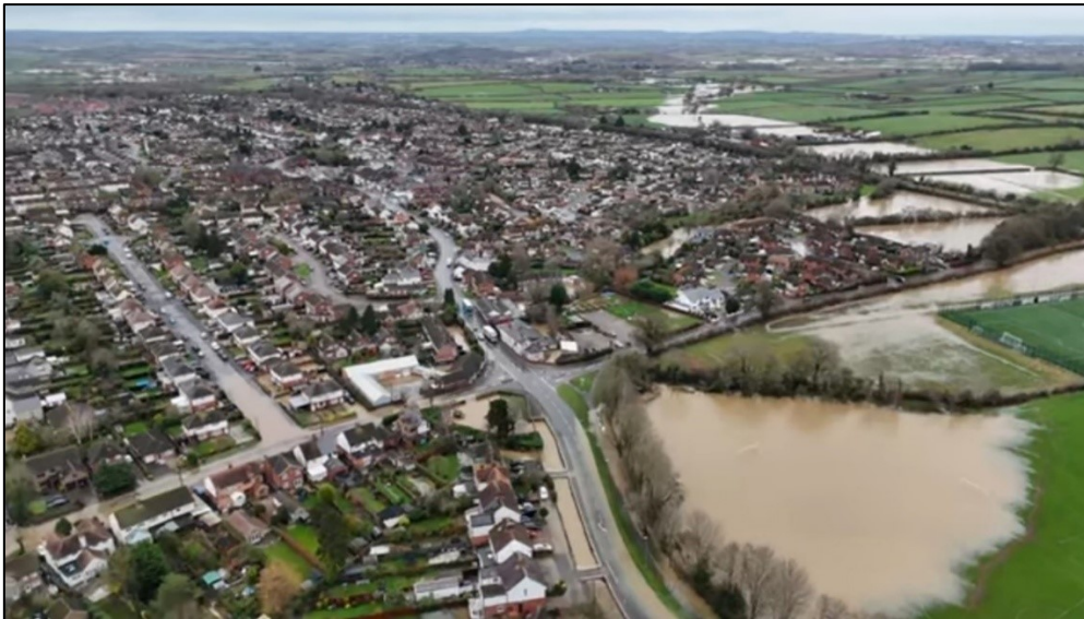
Extensive flooding in Broughton Astley (from watercourses and surface water), January 2025
