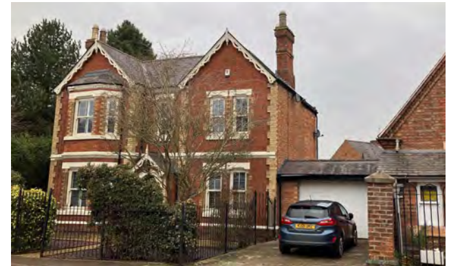
Figure 15: Detailing such as arched brick lintels, decorative brickwork, and original chimney stacks should be retained.
