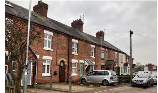
Figure 12: Traditional red-brick terraced houses, featuring arched brick lintels, chimneys, and a strong street frontage.
