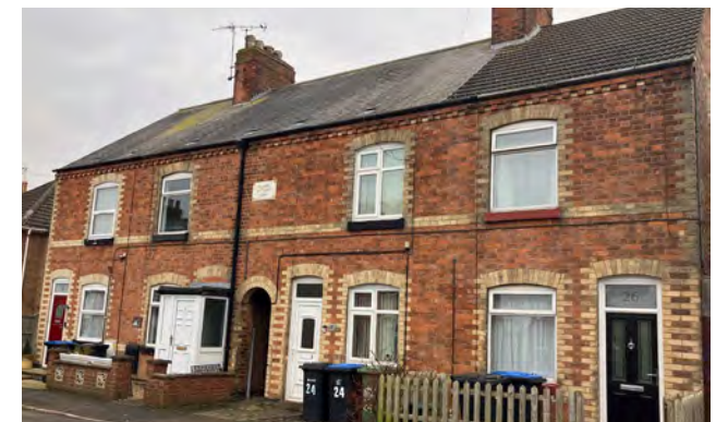
Figure 13: Late 19th-century terraced houses with decorative brick detailing, original chimneys, and uniform building line
