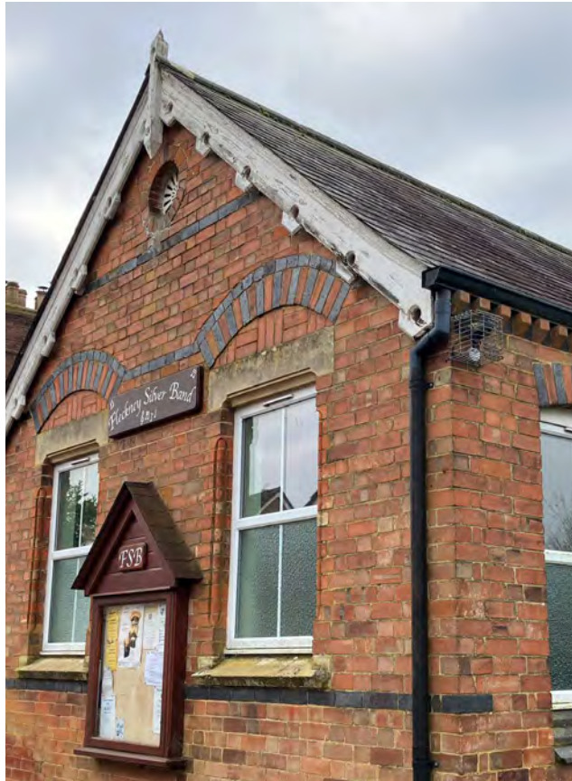
Figure 16: Detailed brick works on traditional buildings
