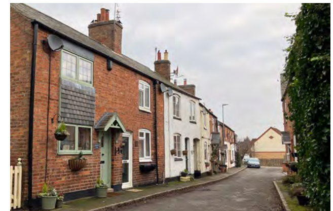
Figure 07: Consistent roof lines of historic cottages create a cohesive built form.
