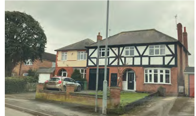
Figure 14: Timber framed structure setback from the road with front gardens and driveways.
