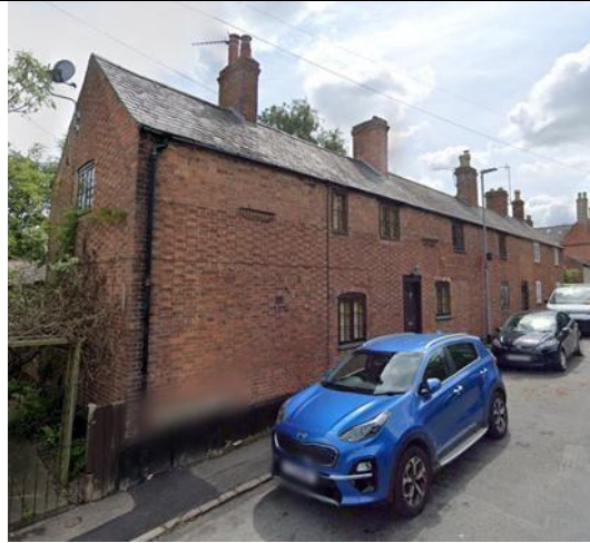
1-3 Scruptoft Rise. A row of chequered red brick cottages in Flemish bond. Of note are alterations to the roof, which changes from an original steep pitch to a wider full second floor
