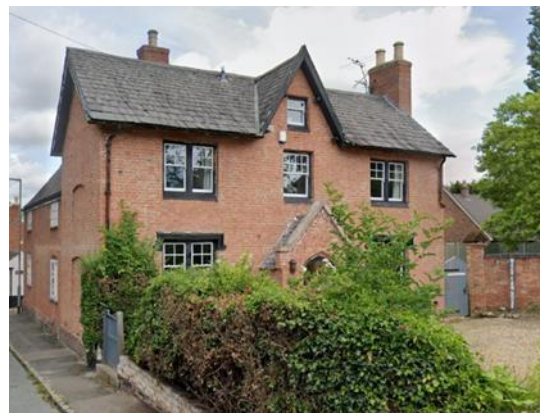
Manor Farmhouse, Stocks Road. The ground floor windows include square 'dripstones' a regional vernacular feature - and 'blind windows' on the western gable
